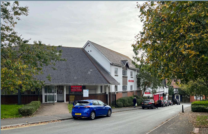
Figure 11 - Oakdale medical centre
