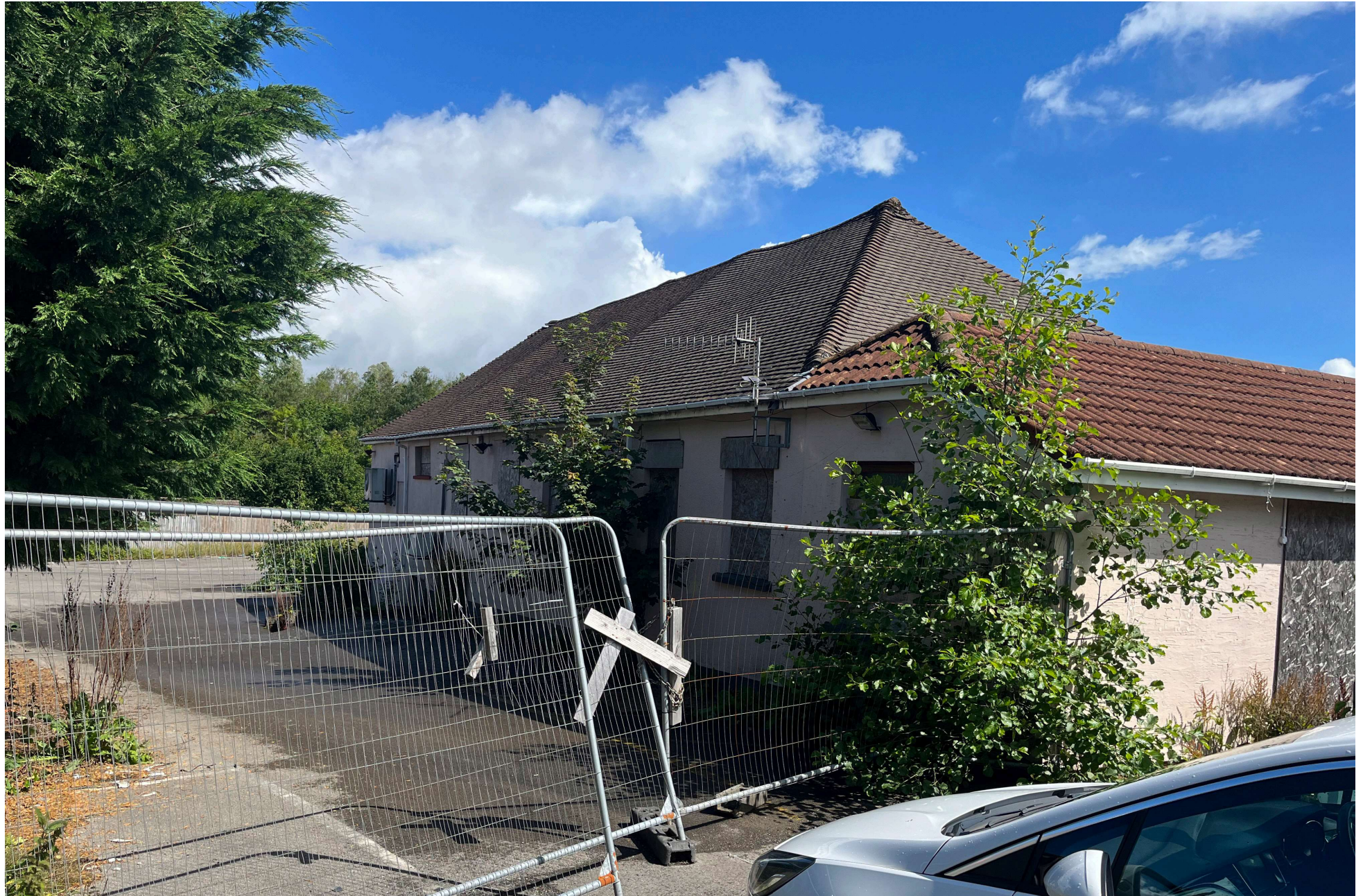
Figure 4 - The former New Forge and existing car parking area to the rear
