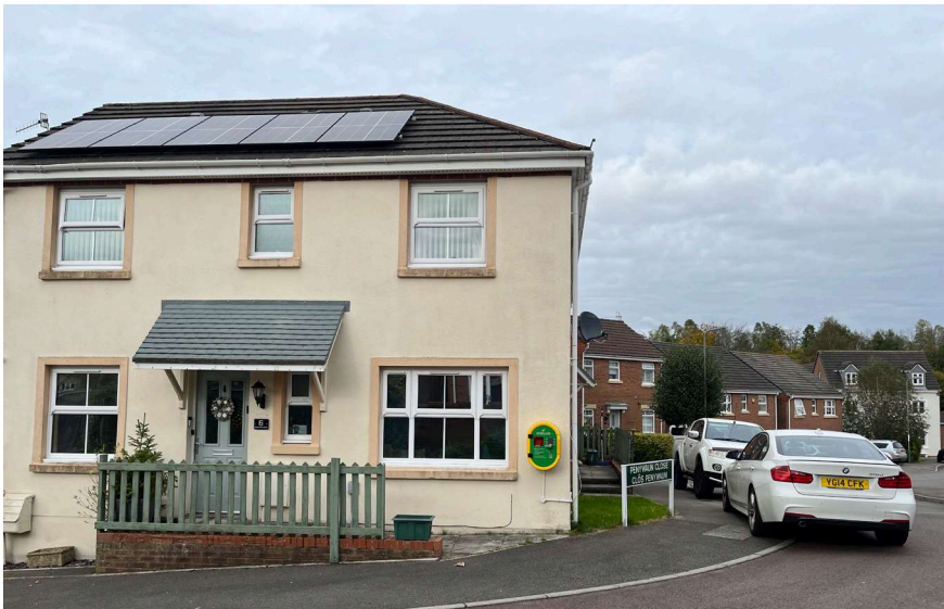
Figure 7 - Dwelling at Penywaun Close
