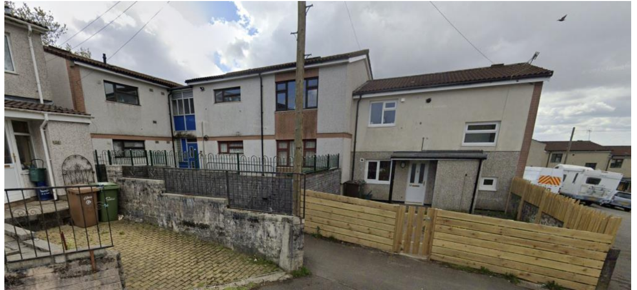
Nearby apartments same building type as per GYR CRC prior to conversion and re-roofing
