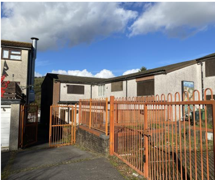
Existing vehicle and pedestrian access to GYR CRC from Grays Gardens
