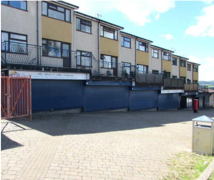
Adjacent vacant retail units
