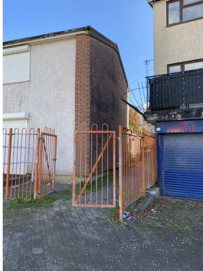
GYR CRC viewed in context with disused Chip Shop
