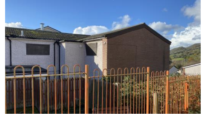
Rear flat roof lift enclosure for demolition
