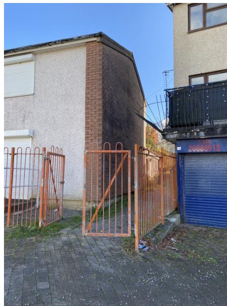
Pedestrian access to GYR CRC from Penllwyn Walk
