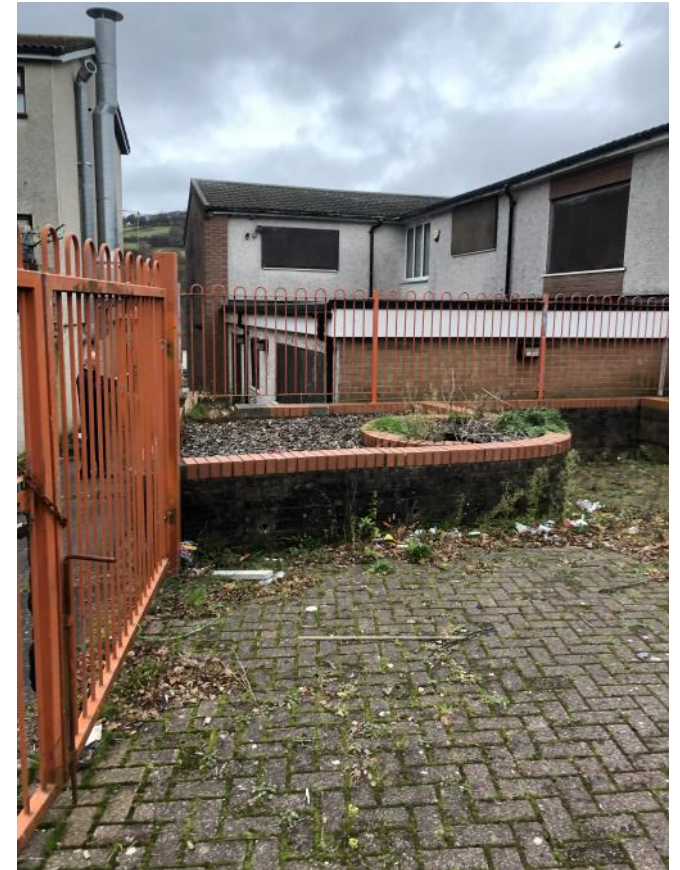
Flat roof extension for demolition
