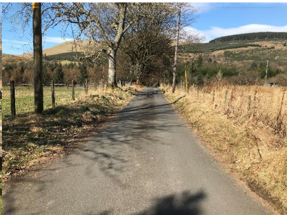
Figure 3: Private Access Road
