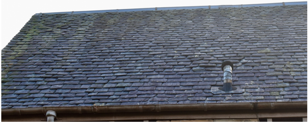
2. Close-up. North facing elevation.
