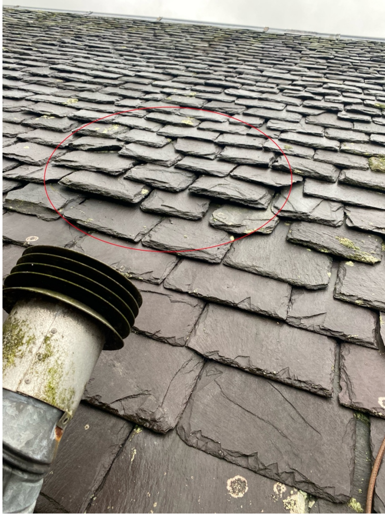
6. North facing elevation. Illustrative roof state.
