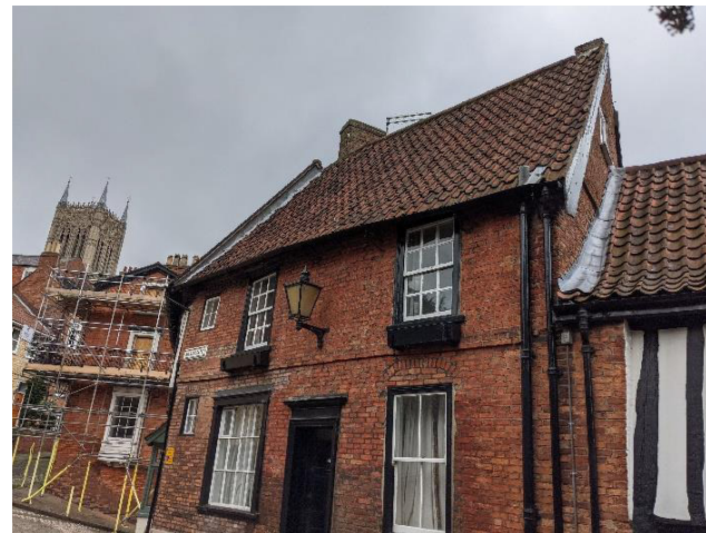
Figure 2: The front elevation of 42 Michaelgate with a view of Lincoln Cathedral on the horizon to the left.
