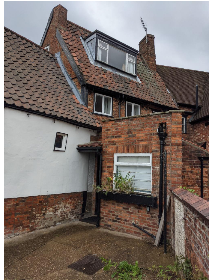
Figure 19: The rear southern elevation of 42 Michaelgate, a single storey flat roofed extension constructed in red brick laid in stretcher bond can be seen in the foreground of the photograph. A casement window with a single top window has been inserted into the southern face of the extension. A 20th century casement dormer window has set into the pantile roof. Two 20th century casement windows can be seen on the first floor. A covered porch and access to the building can be seen to the left of the extension.
