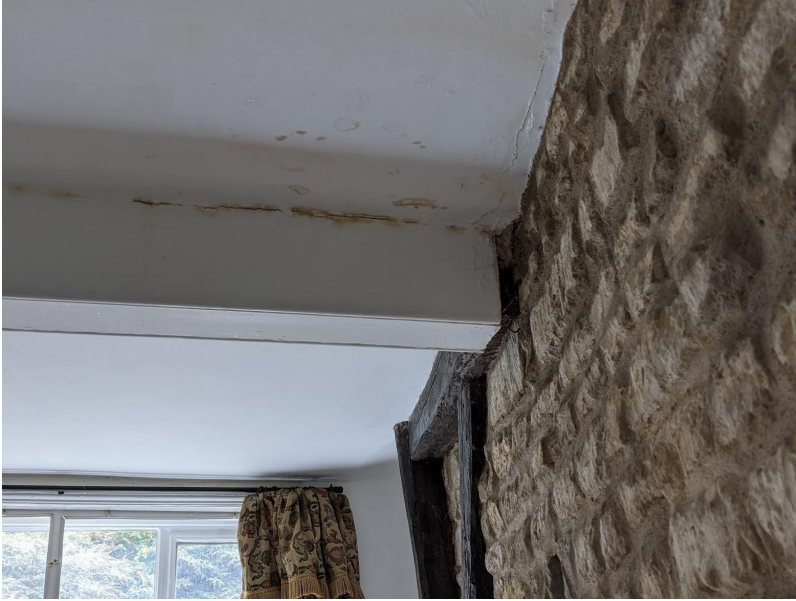
Figure 22: The intersection of the covered ground floor, first floor supporting, timber beam with the 18th century coursed stone wall on the eastern elevation.
