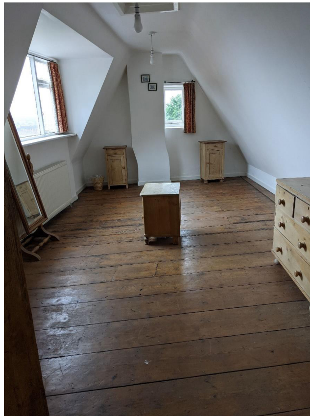
Figure 32: Second floor bedroom, not the curved chimney breast on the southern elevation and dormer window on the left-hand side. The room has a possible 18th century floor, the wide floorboards are possibly 18th century in origin.
