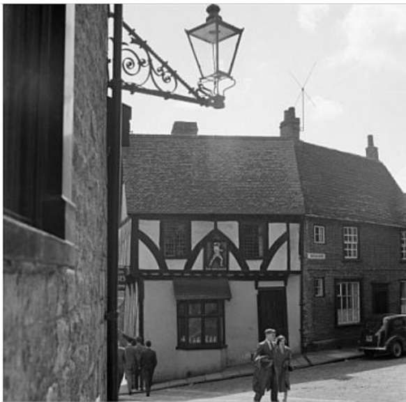
Figure 12: A photo of 42 Michaelgate and Harlequin (right to left) taken in 1961 from Steep Hill. 42 Michaelgate's original chimney stacks can be seen on the south-west gable and eastern gable, both complete with chimney pots.
