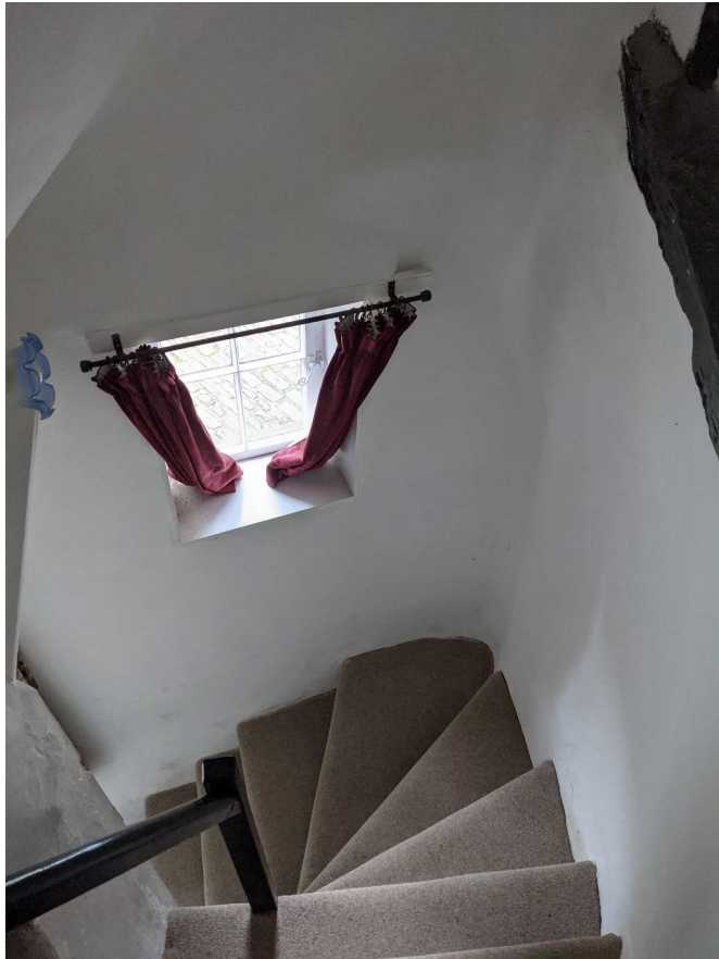
Figure 25: The ground floor to first-floor stairwell and interior view of the first-floor 18th century casement window. Note the slanting party wall with the Harlequin on the right hand side of the photograph. Part of the timber frame can be seen in the top right hand corner.
