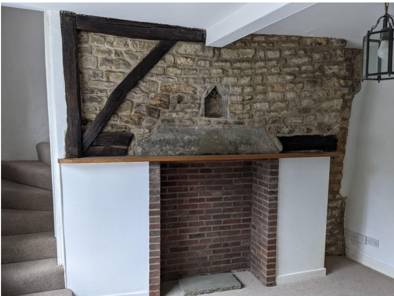
Figure 22: The intersection of the covered ground floor, first floor supporting, timber beam with the 18th century coursed stone wall on the eastern elevation.
