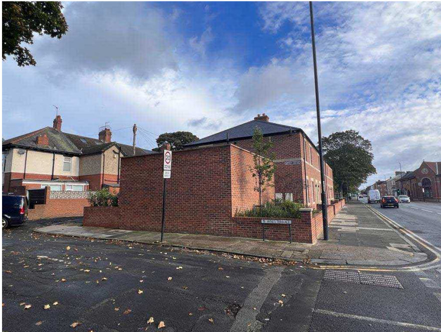
Side Elevation of property from Ayre's Terrace.
