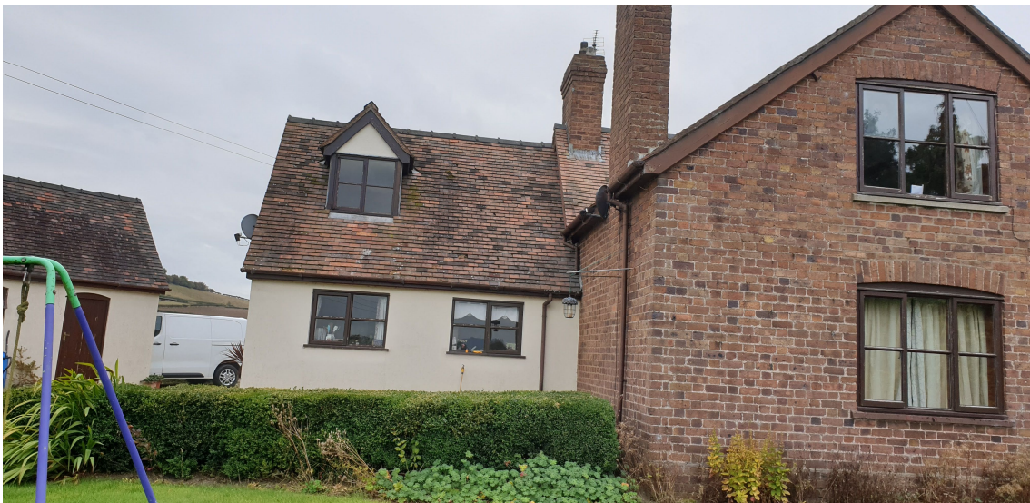
View of East elevation the 1980'S extension will be obscured by the new extension.
