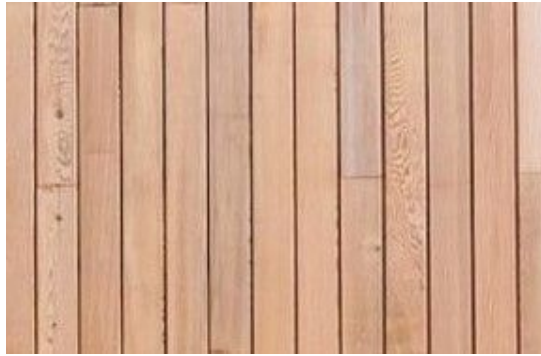
Vertical Douglas fir boarding.
