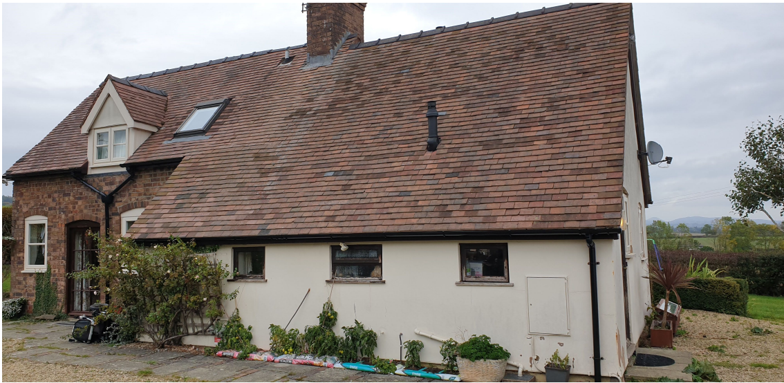
West elevation with proposed extension to the right taken off the 1980's extension.
