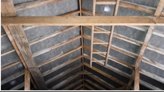
Photo 8 View of close up of roof structure showing modern rafters and BRM lining
