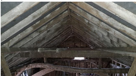
Photo 10 View along rood showing modern roof structure with period hammer beam at bottom of photo
