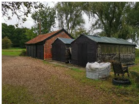
Fig 1: Timber sheds and concrete base
