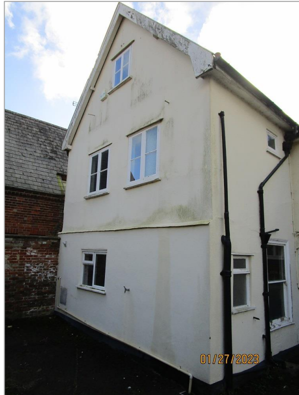
Figs 14 and 15: Second gable on rear of front range of no. 12 (left), also with first floor 4-over-8 sash. Alongside is a 6-over-6 sash (not visible in this photo) and below is a C19 plate glass sash. Fig 15 shows the gabled rear wing of no. 12, with a mixture of C19 sashes and casements and C20 windows. Older maps show rear additions (probably only single-storey) attached to this part of the building.
