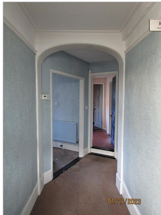
Fig. 16: The ground floor entrance hall of no. 12 has a late Georgian character, overlaying the earlier timber frame (here visible in the beam spanning from front to back, top right). There may be original studwork in the wall to right. Beyond the shallow archway is a modern splayed partition, with the kitchen area beyond and the stair to left.
