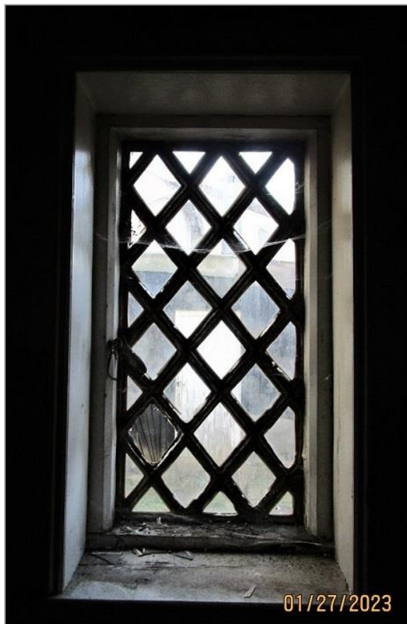
Fig. 36: Lattice casement window in ground floor WC
