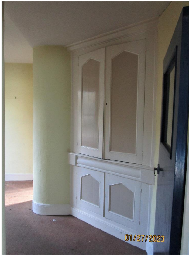
Fig. 24: C19 corner cupboard in space giving off rear ground floor room of front range
