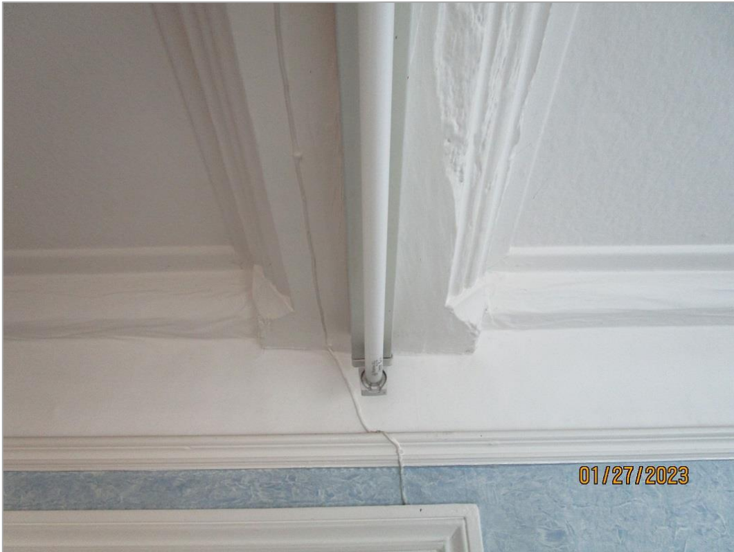
Fig. 18: Detail of C17 beam in room to left of entrance hall
