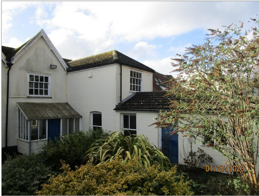
Fig. 13: Rear elevation of no. 14, with single-storey C19 service range to right. This links to the brick C18 rear range, of brick with hipped roof (now covered, like the whole of the rear elevation, with concrete tiles). The C18 range has a first floor 4-over-8 glazing bar sash, while on the ground floor flank elevation is a C19 plate glass sash. Above this sash, the scar of the flashing of the full-width conservatory shown on the old maps can be discerned. This conservatory has been replaced by a small conservatory to no. 14 only. The rear elevation of the front range is timber framed and gabled, with bargeboards and 4-over-8 sash at first floor level.
