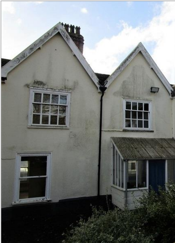
Figs 14 and 15: Second gable on rear of front range of no. 12 (left), also with first floor 4-over-8 sash. Alongside is a 6-over-6 sash (not visible in this photo) and below is a C19 plate glass sash. Fig 15 shows the gabled rear wing of no. 12, with a mixture of C19 sashes and casements and C20 windows. Older maps show rear additions (probably only single-storey) attached to this part of the building.
