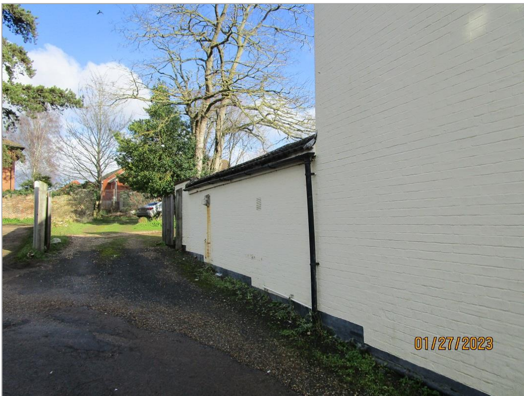
Fig. 12: Beyond the C18 rear range is a single-storey C19 service range, also of painted brick and with a concrete pantile roof. It presents a blank face to the side approach.
