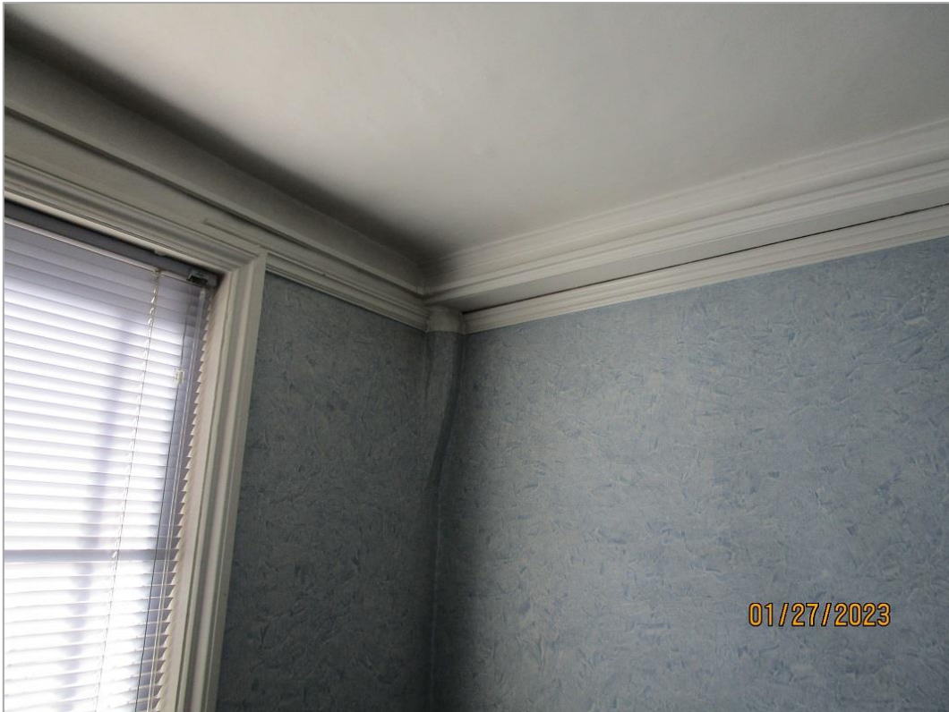
Fig. 20: A papered-over jowled post in the southwest corner of the room to right of entrance hall
