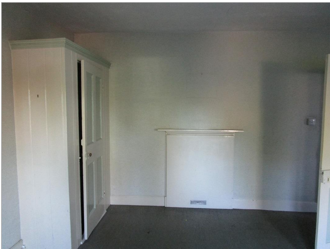
Fig. 27: C19 cupboard and blocked fireplace, rear wing first floor
