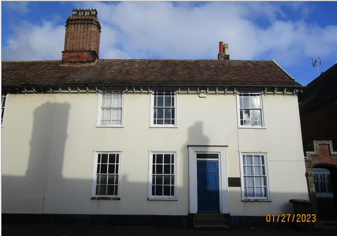
Fig. 9: Front elevation of no.12. The large central stack with saw-tooth brickwork and the steep tiled roof are the only obvious pointers to the building's C17 origin. The present appearance is largely of mid-C19 character, of three bays plus off-centre door (the panelled door itself a late C20 replacement) with moulded surround, rectangular fanlight and stone steps. Smooth rendered walls, bracketed eaves, flush frame glazing bar sashes with marginal lights.
