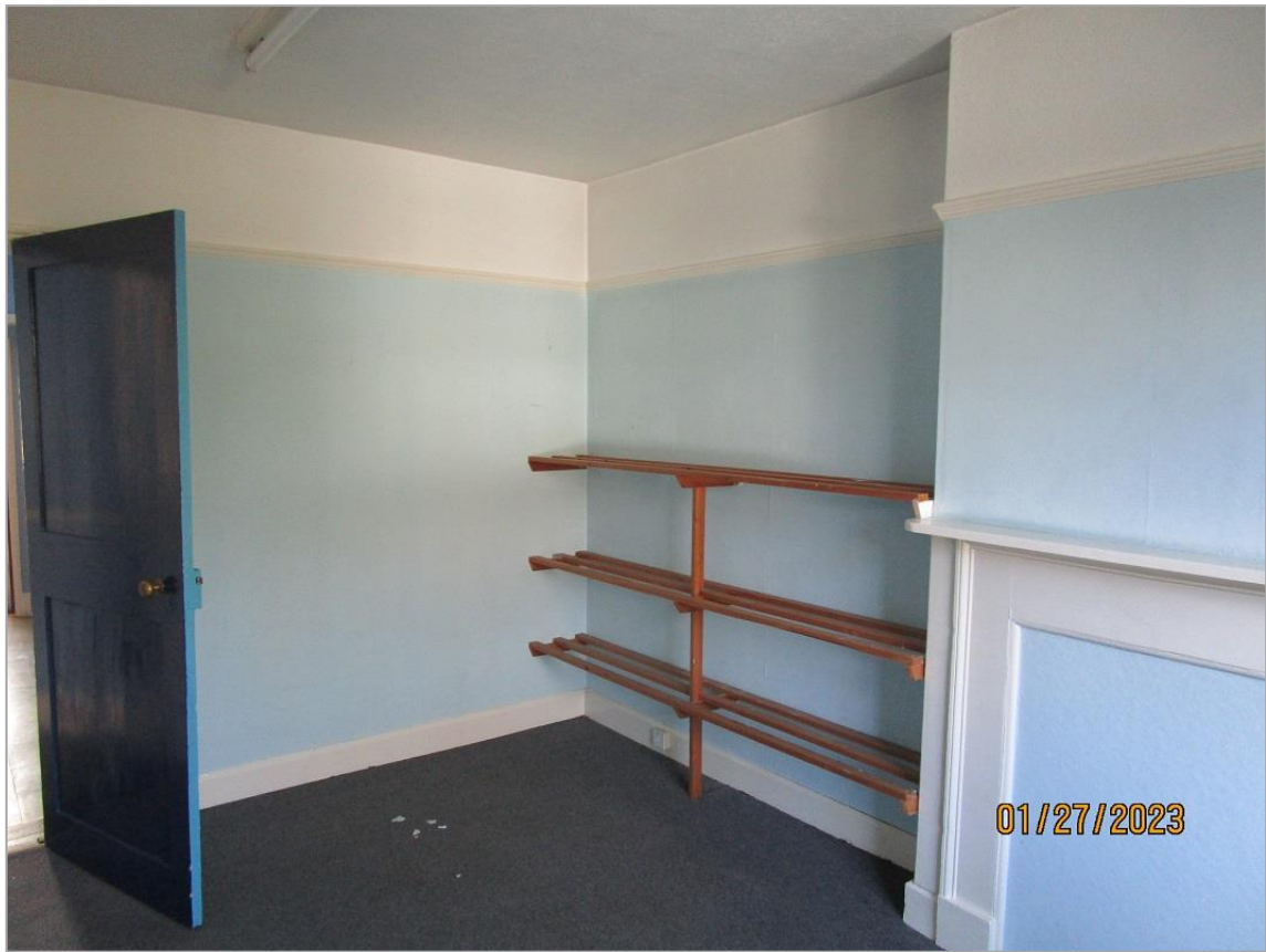
Fig. 39: Two-panel door and boarded-up fireplace in C18 rear range, first floor.
