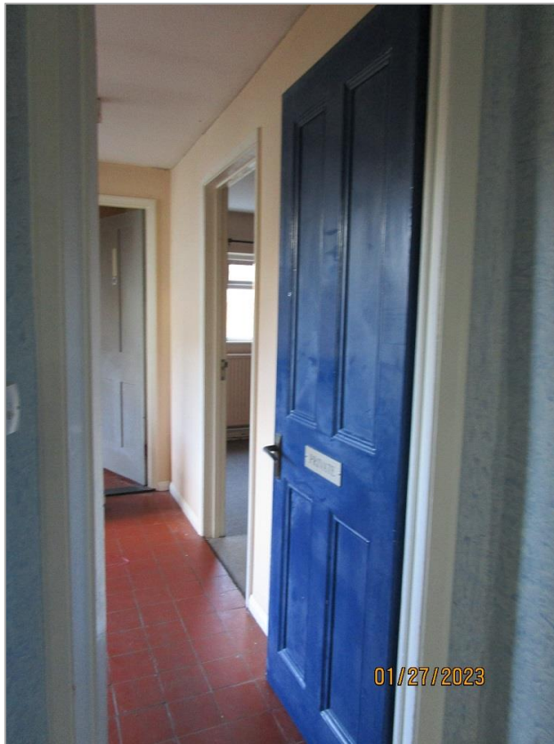
Fig. 25: Door to ground floor rear range, where there is a raised (tiled floor). The kitchen area has modern partitions and no visible historic features or finishes.
