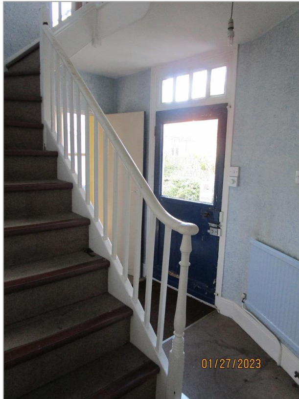
Fig. 22: The stair to first floor is of late C18 or early C19 character, with closed string, square balusters, turned newel and moulded handrail, all painted.
