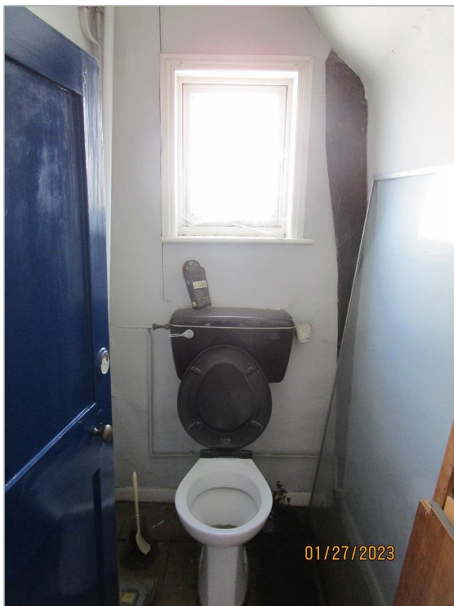
Fig. 41: Two-panel and exposed post in first floor WC.
