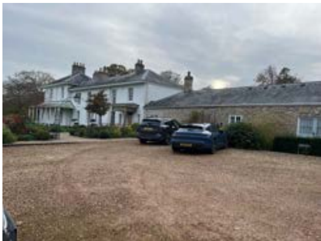
Picture 1: Looking west towards main house with service range on the right
