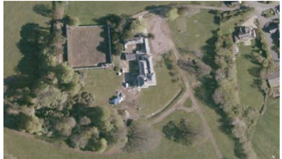
Figure 23: 2010 Aerial shows planning approval 10/0975/LBC being implemented. Note: the kitchen garden has been cleared ready for conservation.
