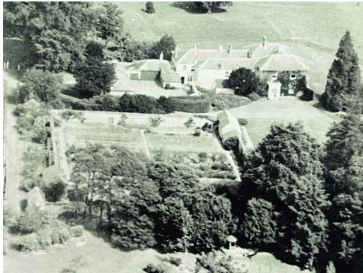
Figure 25: Offwell House c1900 shows the original driveway at the west of the property. Note the original entrance portico which still exists.
