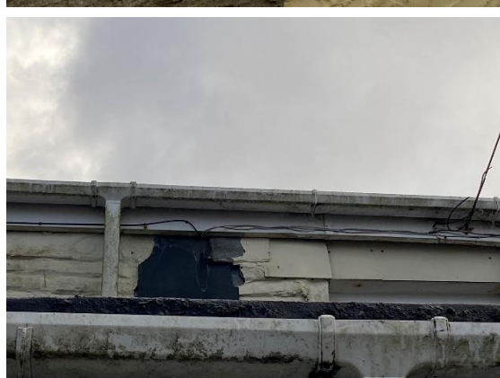
Figure 5: The external gaps present on the former pub including gaps under roof and hanging slates, gaps into the wall and underneath fascias.
