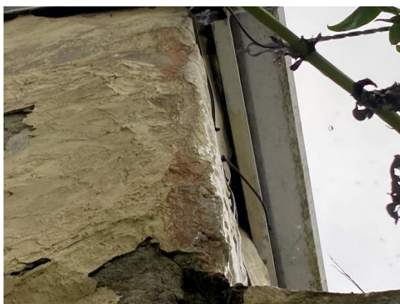
Figure 5: The external gaps present on the former pub including gaps under roof and hanging slates, gaps into the wall and underneath fascias.
