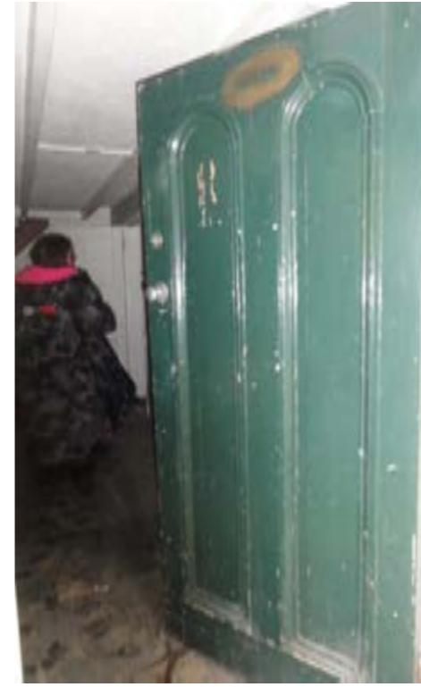
Photo059–Main House Ground Floor
