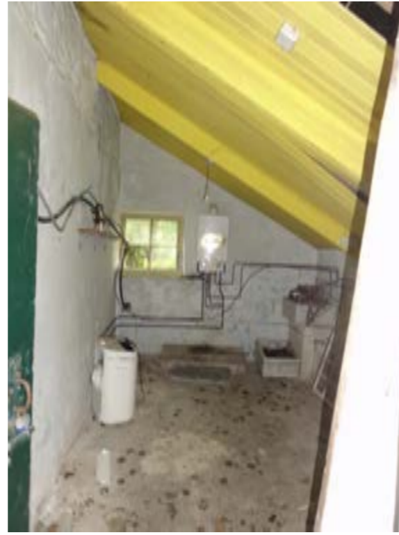
Photo058–Main House Ground Floor
