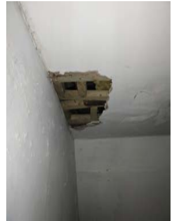
Photo072–Main House Ground Floor
