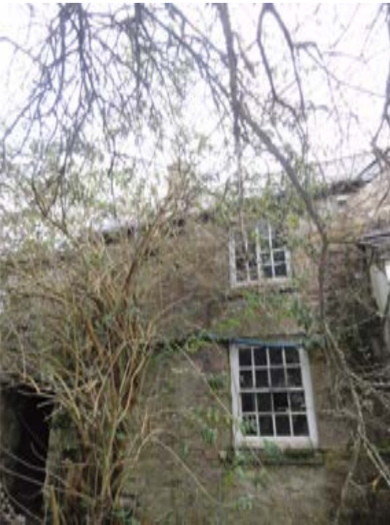
Photo061–Main House Ground Floor
