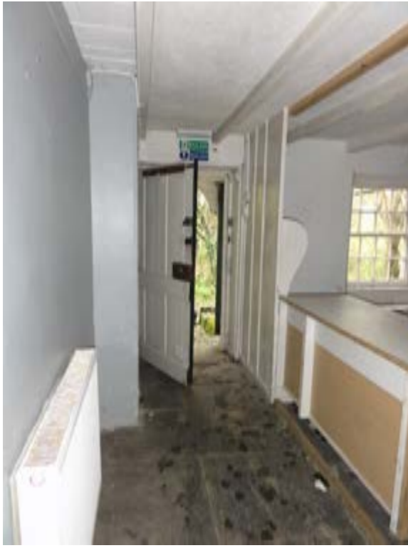
Photo065–Main House Ground Floor
