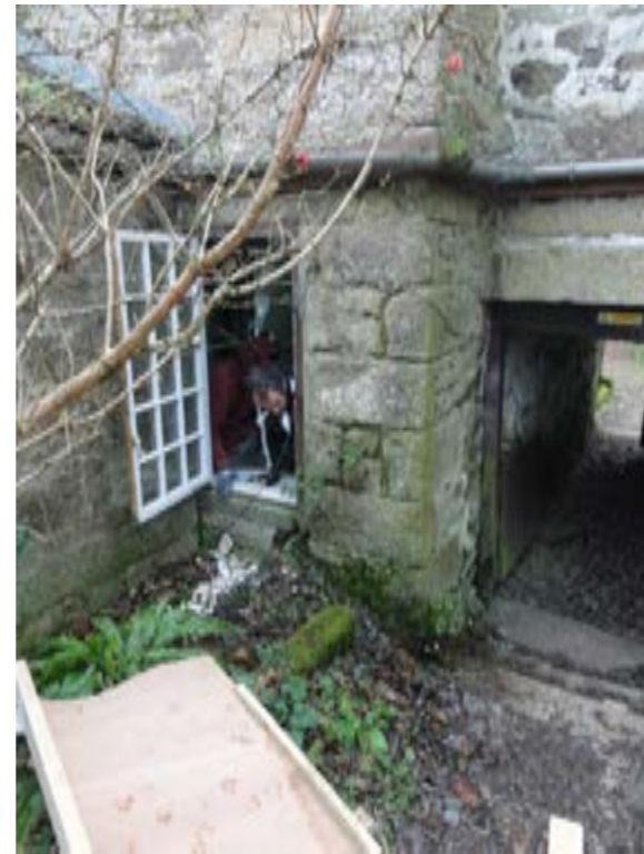
Photo070–Main House Ground Floor
