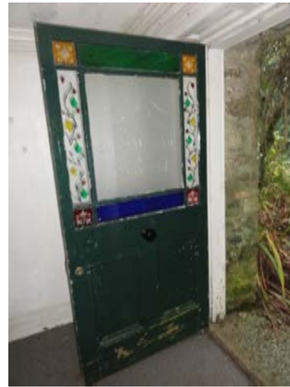
Photo075–Main House Ground Floor
