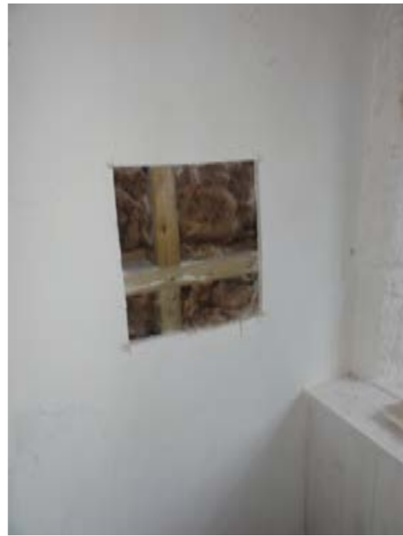
Photo074–Main House Ground Floor
