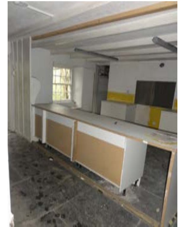
Photo064–Main House Ground Floor
