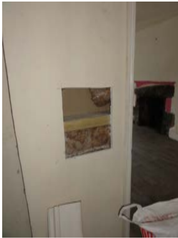
Photo073–Main House Ground Floor
