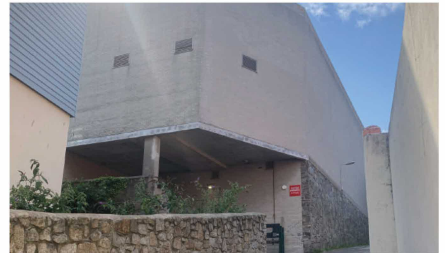
Photo 5: View looking towards the rear of the poundstretcher building
