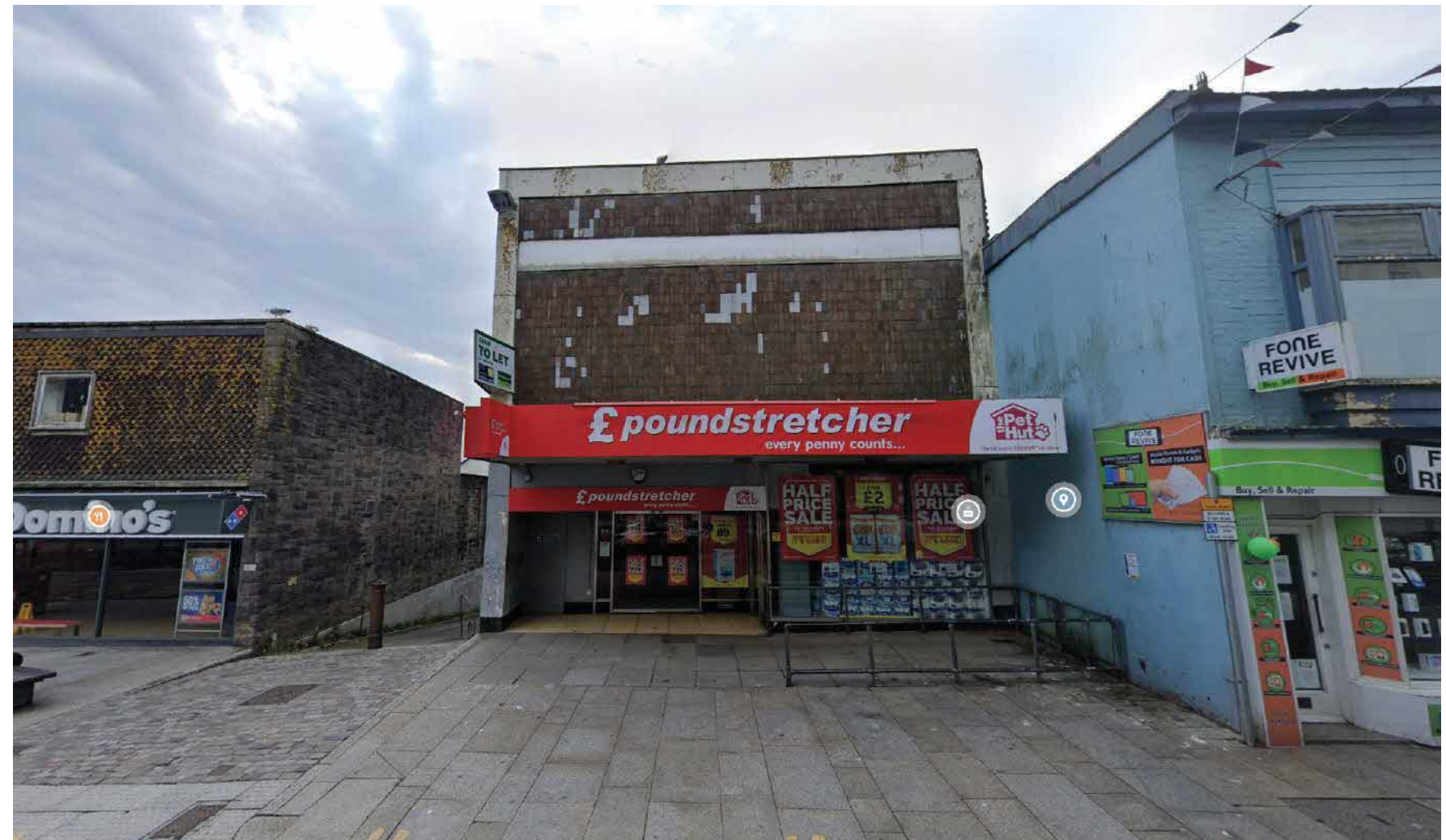
Existing facade of building
