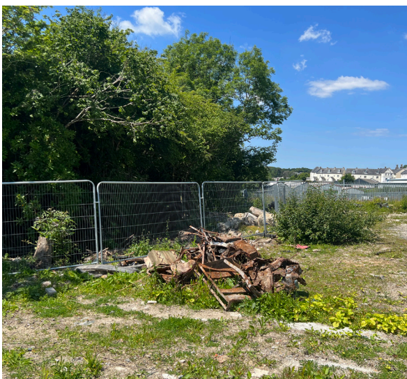
5. On site viewed looking West towards railway embankment
