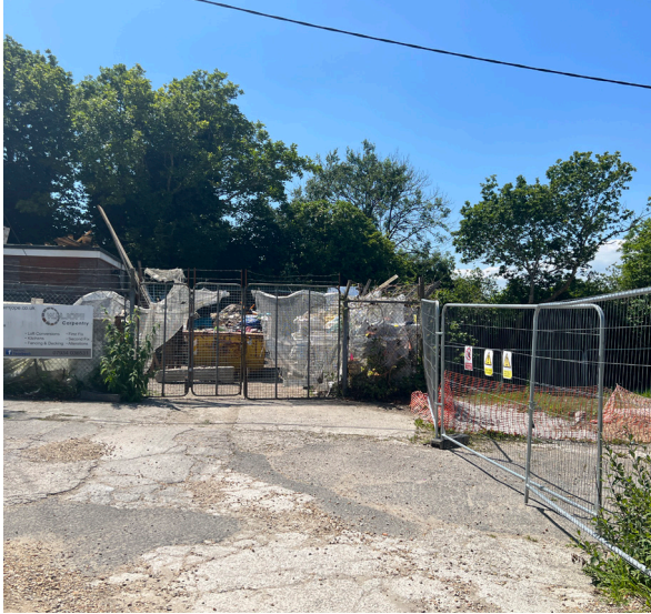
9. Shared site access looking at proposed site entrance
