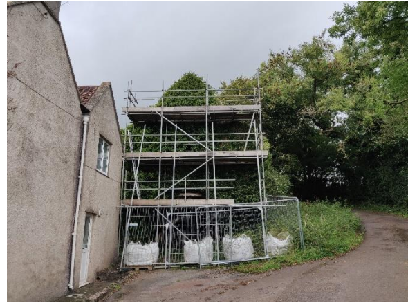
Photo 16. The southern elevation of the Wagon House.
