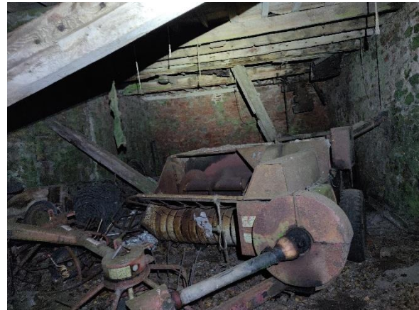
Photo 18. An internal view of the ground floor of the Wagon House (photo taken at night).
