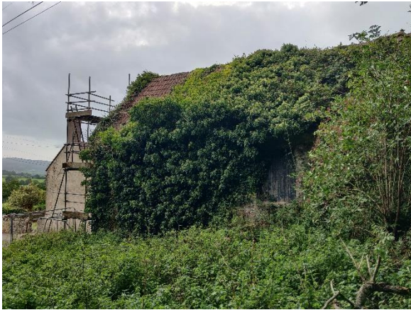
Photo 15. The eastern elevation of Wagon House.
