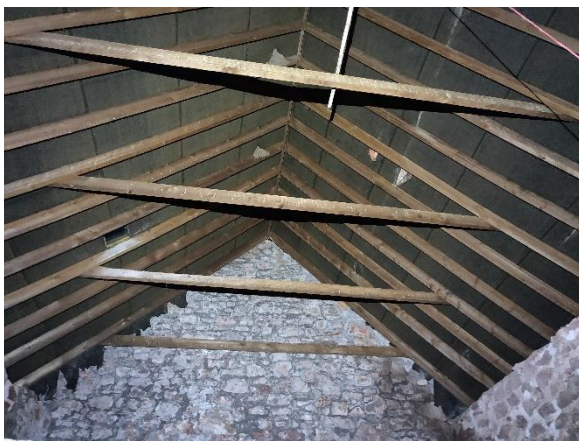
Photo 9. An internal view of the Main Barn.
