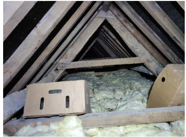
Photo 4. The northern roof void of the Farmhouse.
