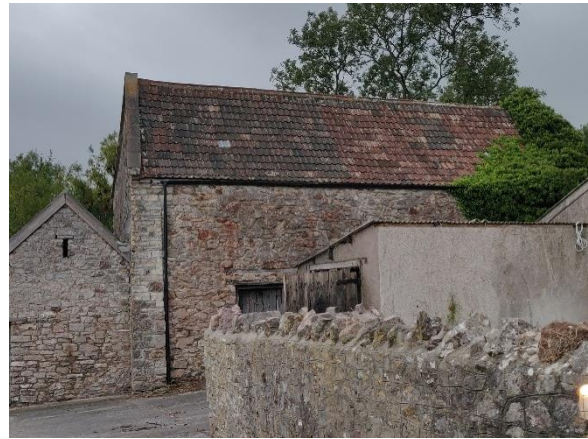
Photo 8. The eastern elevation of the Main Barn.
