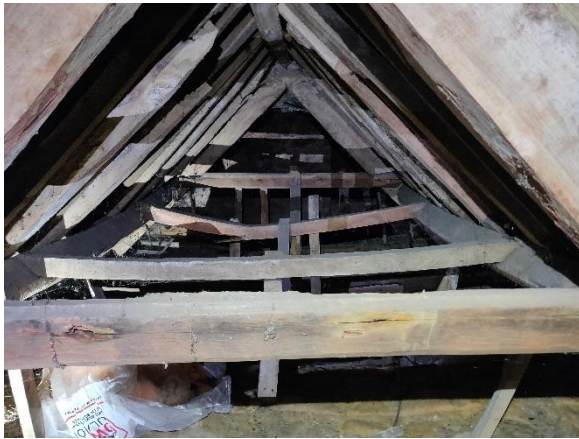
Photo 3. The south-western roof void of the Farmhouse.
