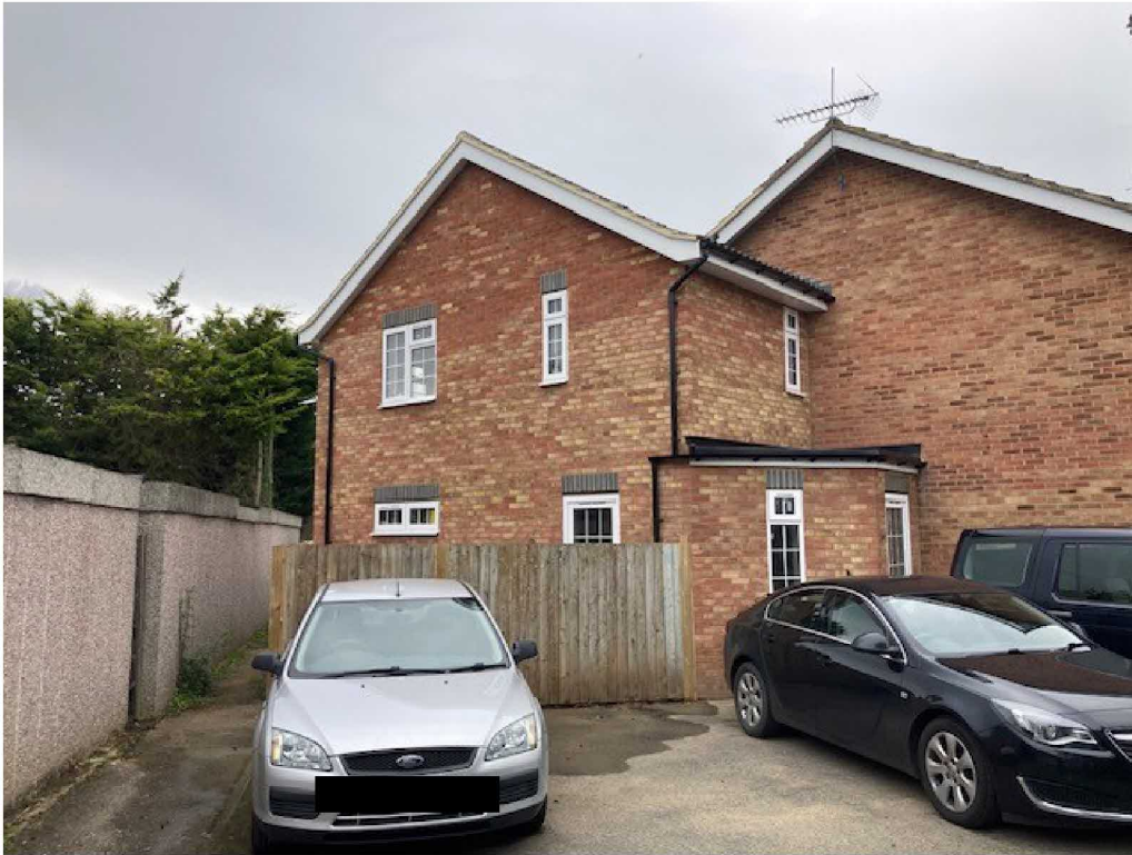
Photo 1 – As-built extension at 7 Krohn Close, Buckingham.
