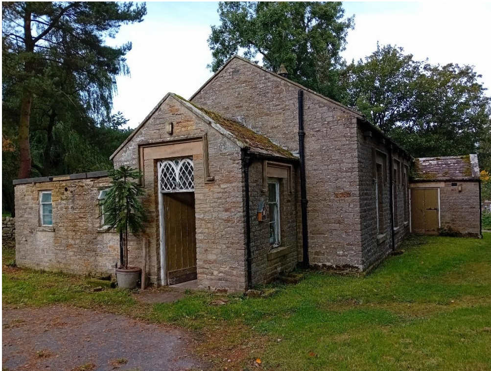
Photo 1 – Church Hall, South Elevation
