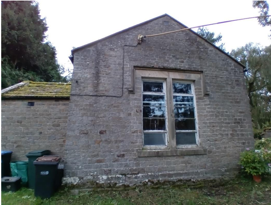
Photo 2 – Church Hall, North Elevation
