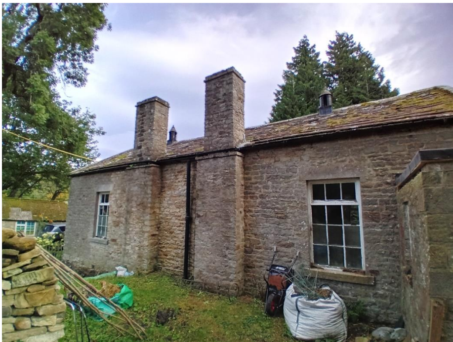
Photo 3 – Church Hall, West Elevation
