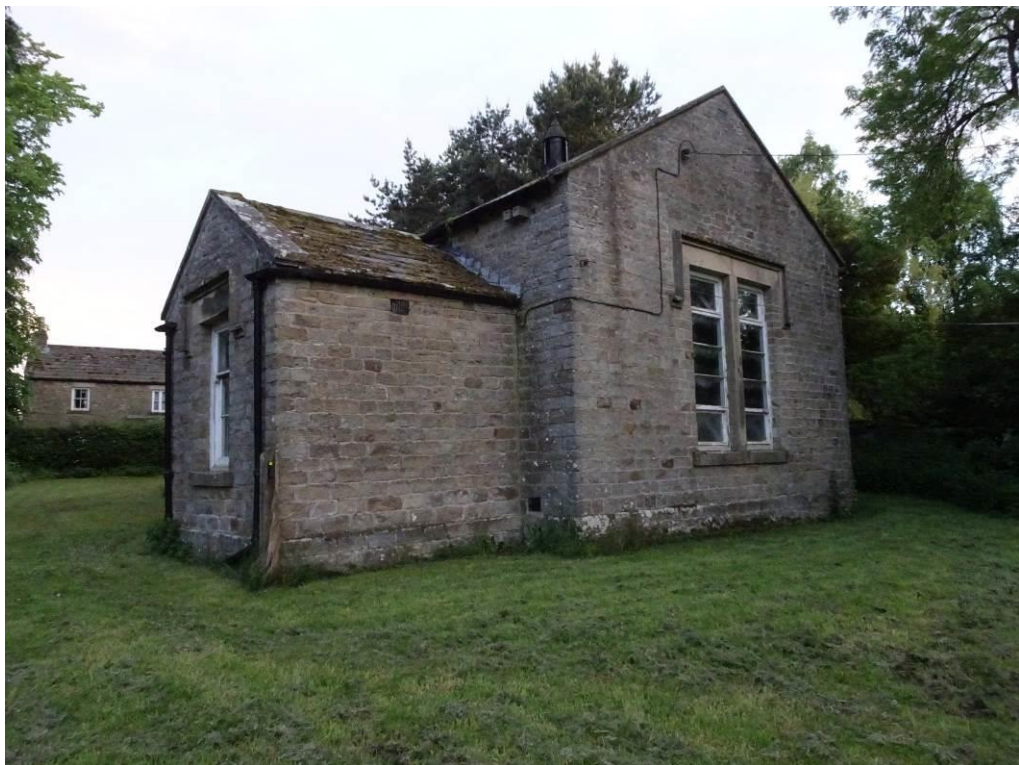
Northern end of building
