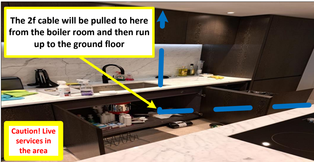
4 Basement Level Kitchen
