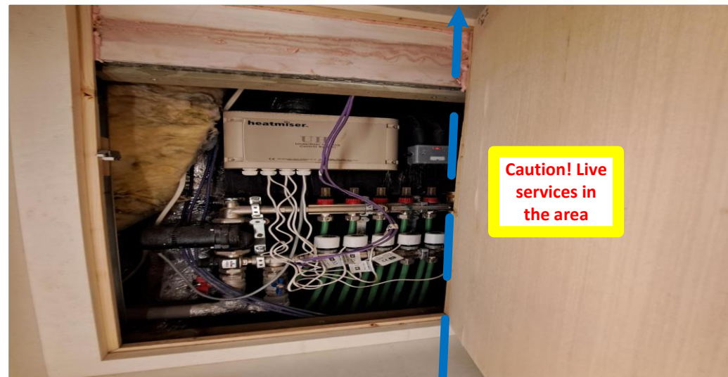
22 2f cable will continue going up to the 7 th floor
