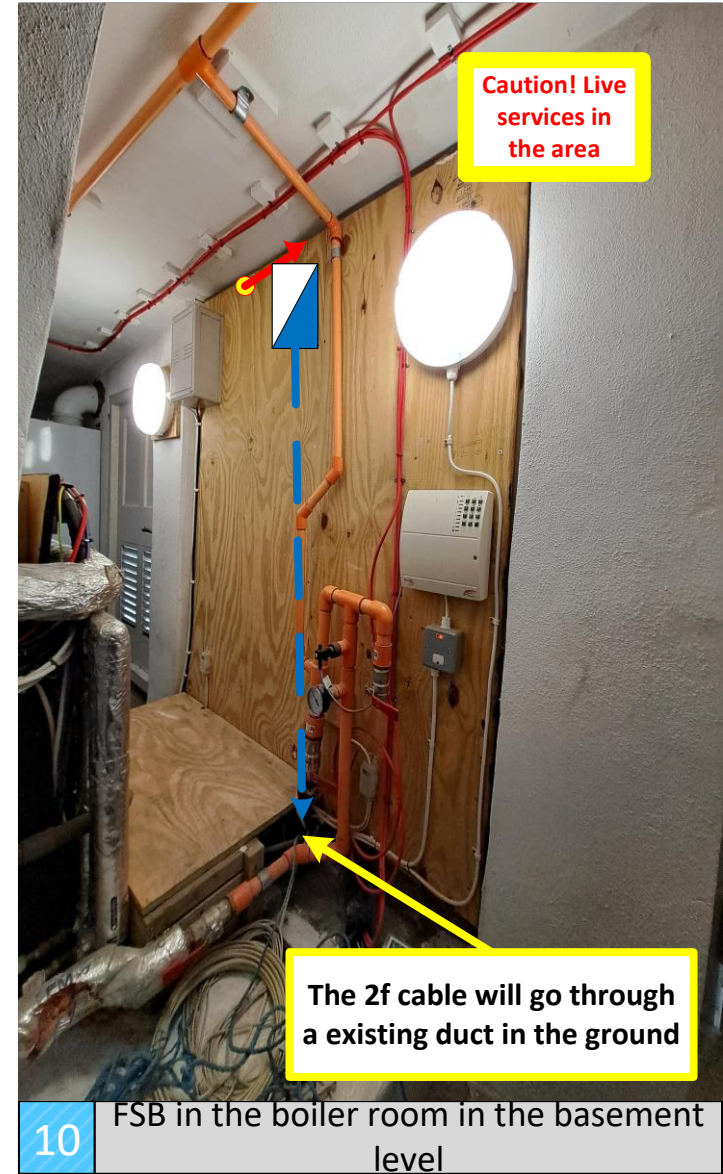
9 12f cable going into boiler room from the basement level
