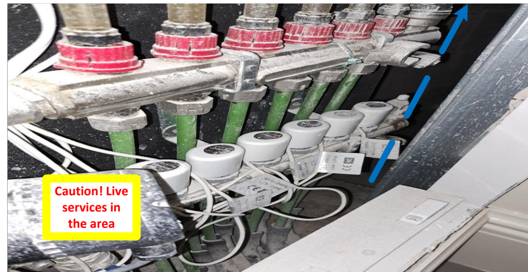
14 The 2f cable will go up to the 1 st floor from the existing access panel in the wall
