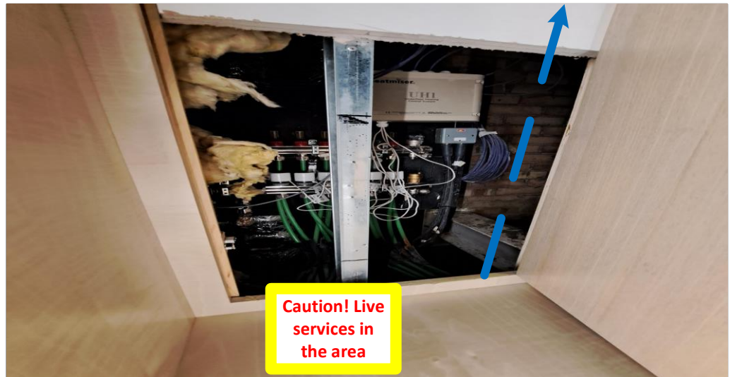
26 2f cable will continue going up to the 7 th floor
