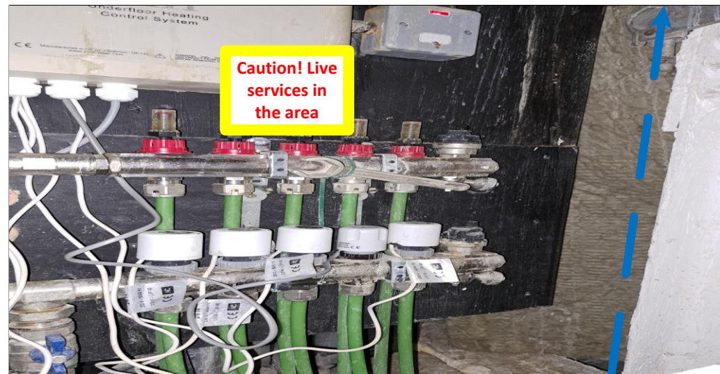
20 2f cable will continue going up to the 7 th floor
