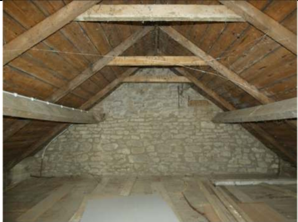
Photograph 14. The partially enclosed roof void above the north bay
