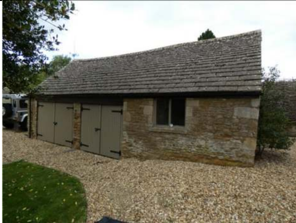
Photograph 1. The west elevation
