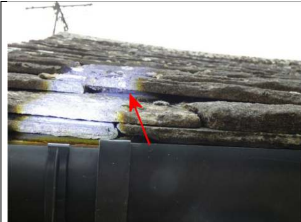
Photograph 7. Further example of an opening under the slates on the west-facing roof pitch
