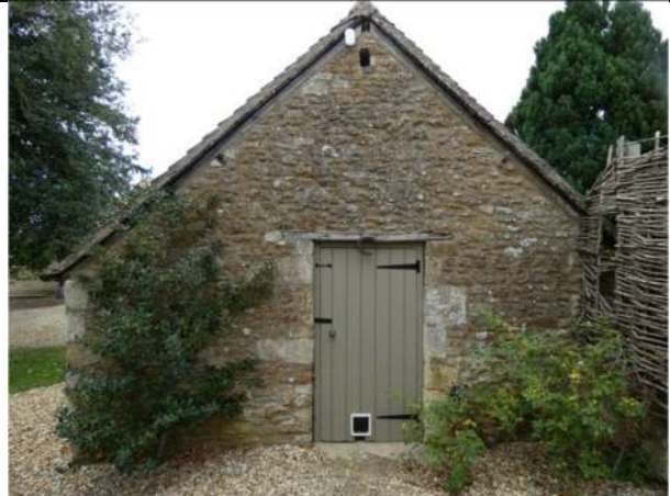
Photograph 2. The south elevation
