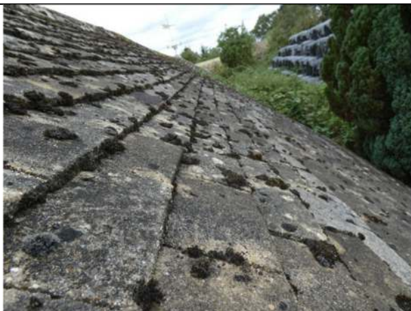
Photograph 5. The sealed east-facing roof pitch
