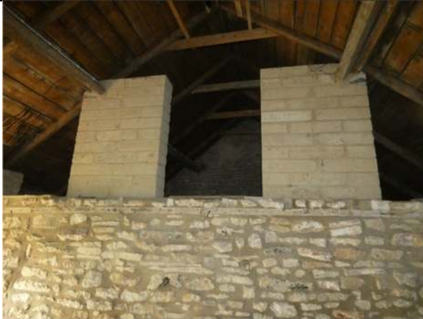
Photograph 13. The interior of the central bay
