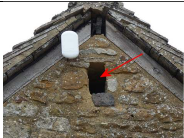
Photograph 4. Opening in the south gable wall
