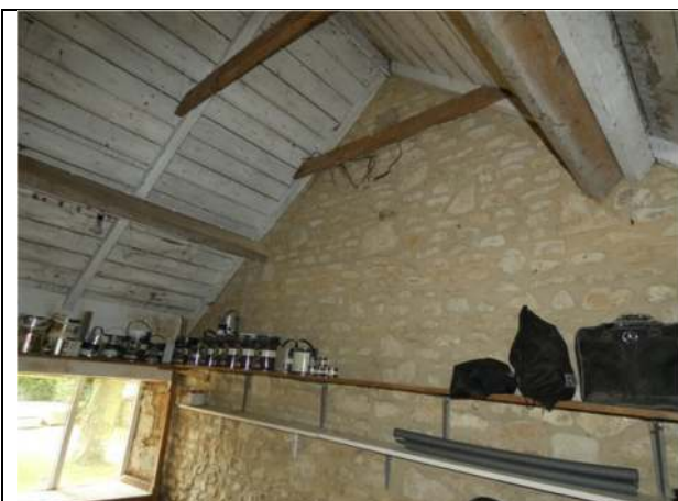
Photograph 11. The room at the southern end of the building
