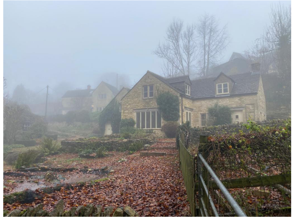
View from the south of the site looking towards Woodside Cottage across mature gardens
