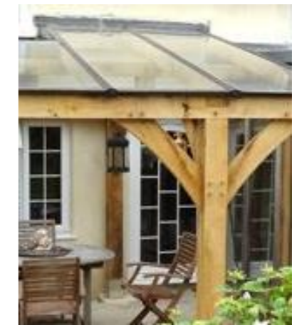
Timber frame porch with metal standing seam roof
