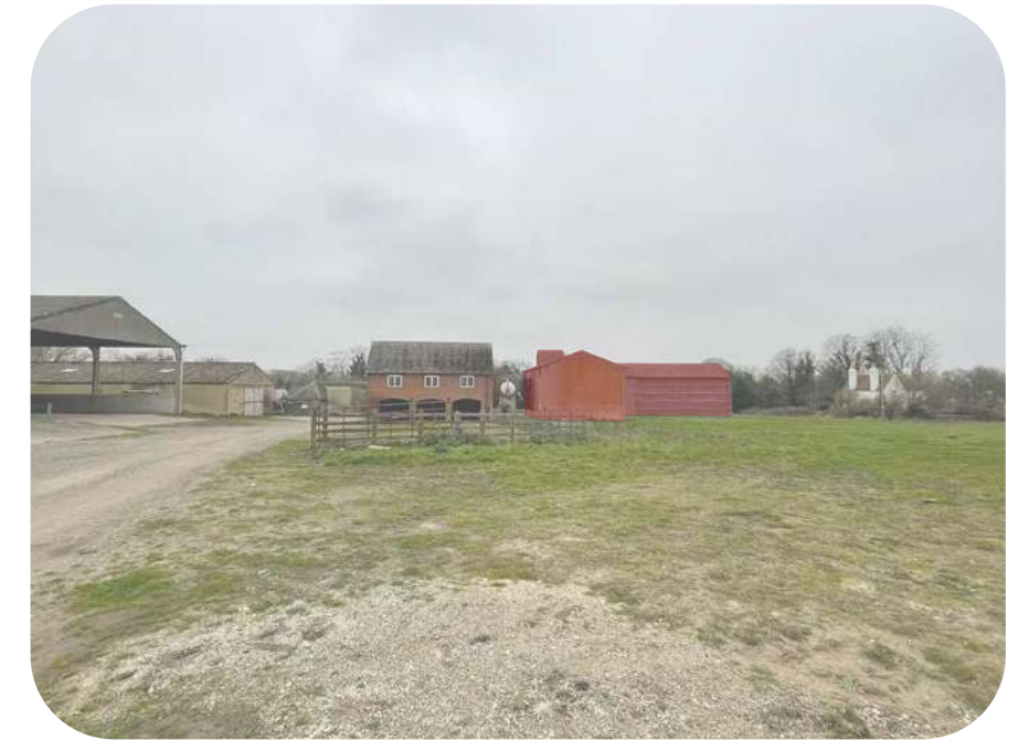
View from east showing proximity of grain store to neighbouring property.
