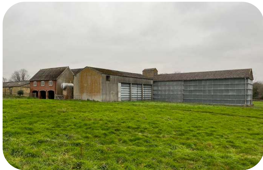
Above - View of Grain Store & Grain Drier shown in proximity to Oast Right - View of Grain Store from north
