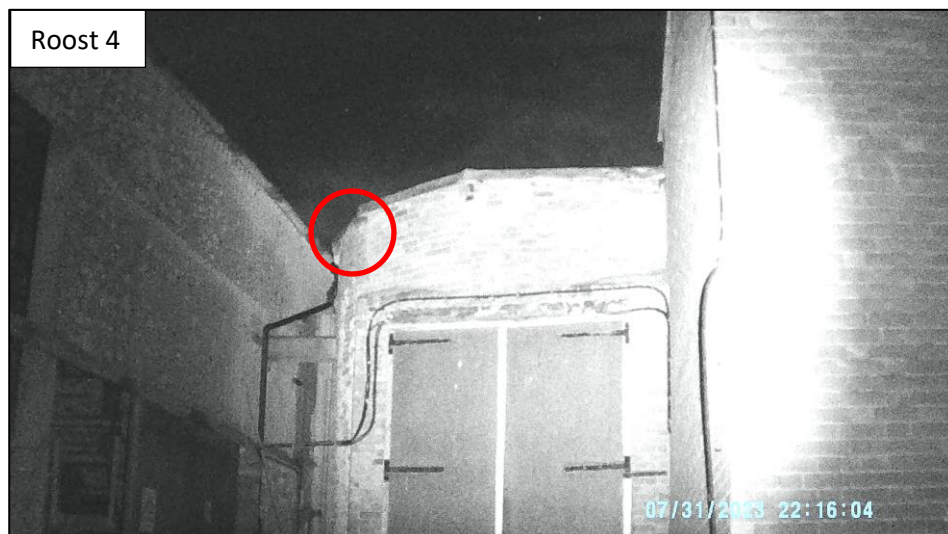
Photo A5.4: Location of emergence point from under felt on 10.07.2023 and 31.07.2023 for Roost 4, common pipistrelle day roost (Building B2, view from IR Whisker camera).
