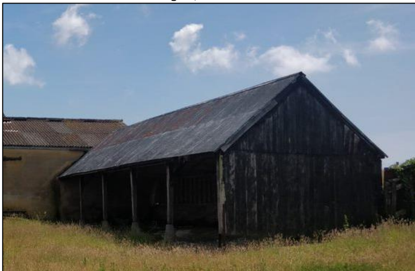
Photo 4.15: Building B4, western and northern elevations
