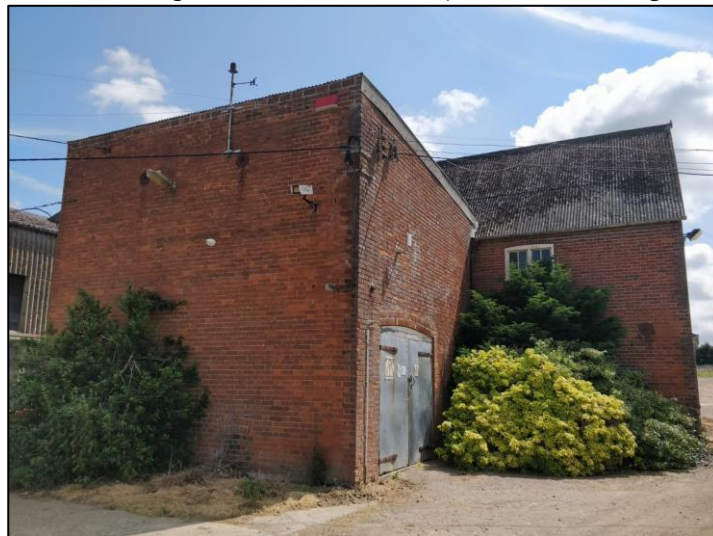
Photo 4.9: Building B2, western elevations (no. 1, 2 and 3 in Figure 4.1 ).
