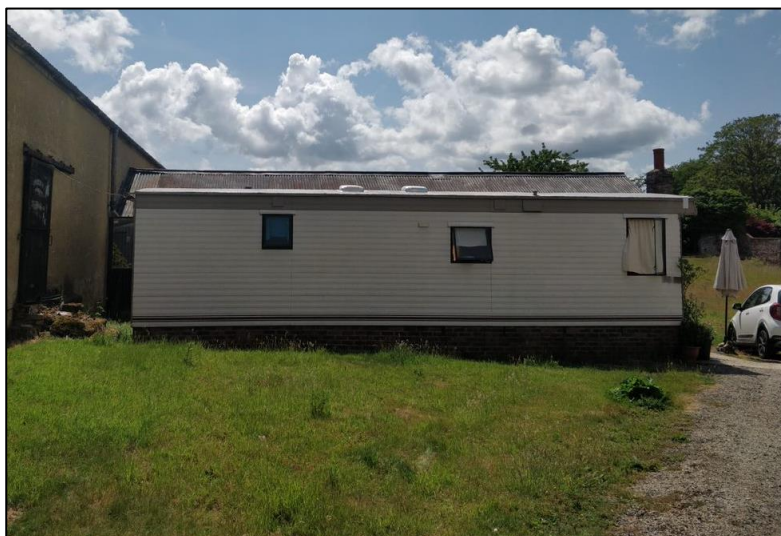
Photo 4.17: Building B6, northern elevation.
