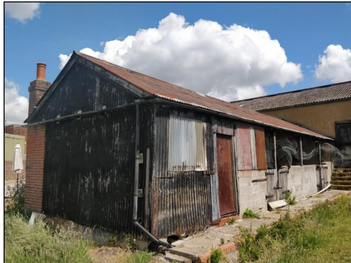
Photo 4.16: Building B5, western and southern elevations.
