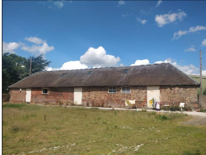
Photo 4.7: Building B1, facing north
