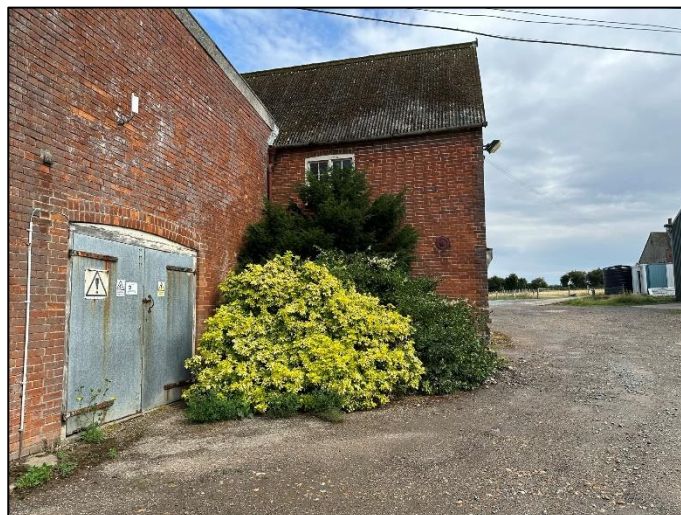
Photo 4.6: Introduced shrub located within the site boundary, facing north-east
