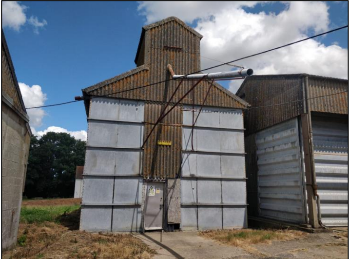
Photo 4.19: Building B8, southern elevation.
