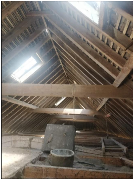
Photo 4.8: Building B1, view of internal loft void form loft hatch
