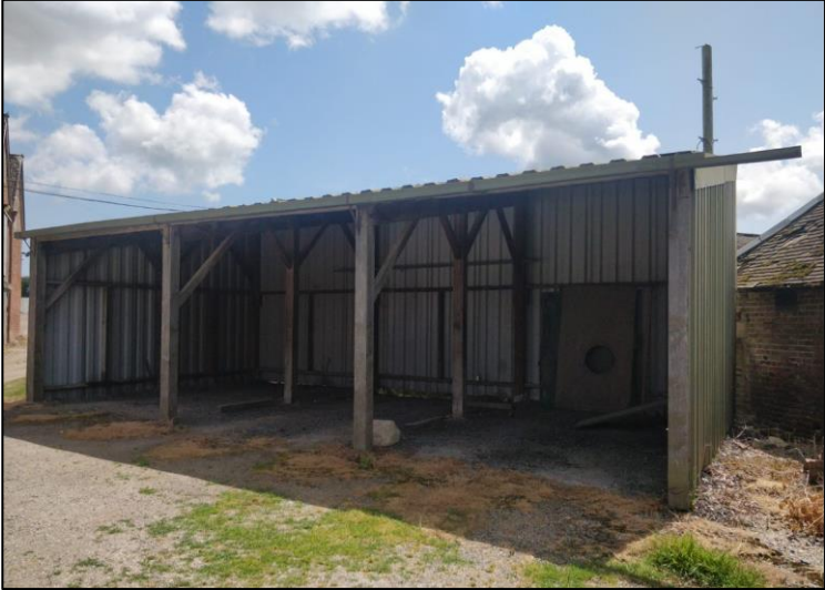
Photo 4.18: Building B7, western and northern elevations.
