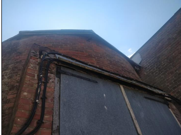
Photo 4.13: Building B2, north-west elevation (no. 7 in Figure 4.1 ).
