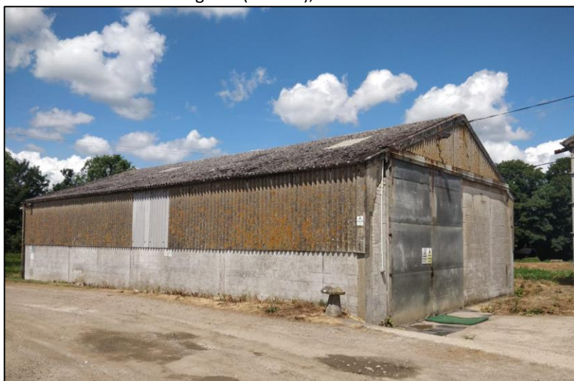
Photo 4.21: Building B10 (off-site), southern and eastern elevations.
