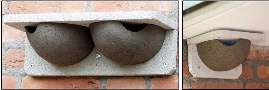
Figure A8.2: Examples of suitable Woodstone, long-lasting house martin nest cups (CJ Wildlife, 2023)
