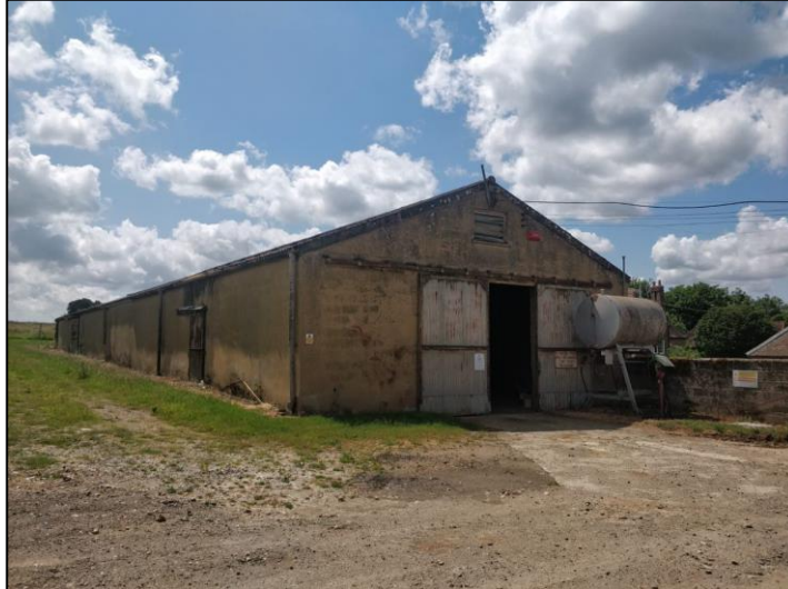
Photo 4.14: Building B3, northern and eastern elevations.
