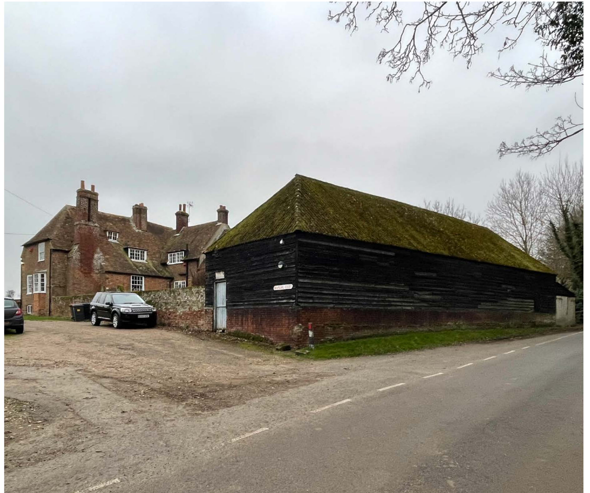
Above: Entrance to Bramling Court Farm showing Grade II listed Bramling Court and locally listed stable building.
