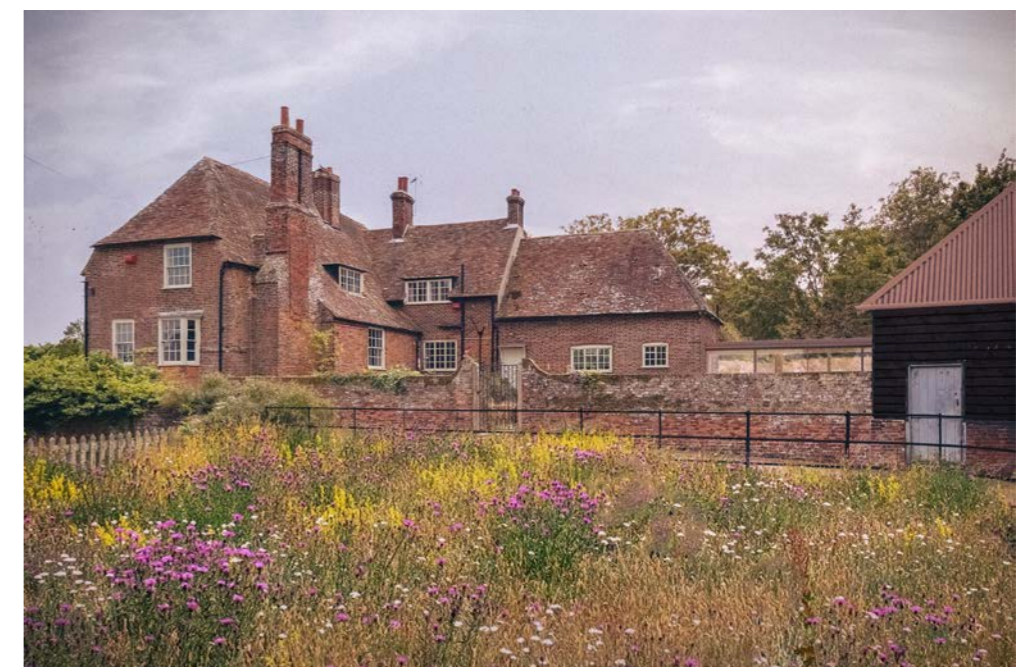
Approved Design - Farmhouse Extension and reconfiguration - View of proposal from site entrance
