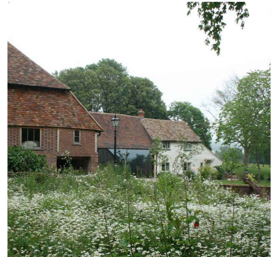
Above: The Hall - Grade II* Listed - Extensive repair, renovation & extension complete
