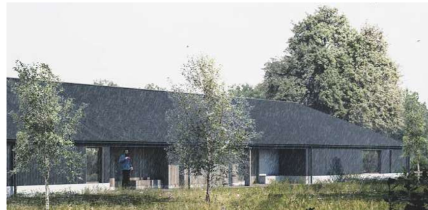
Above: Bossingham Farm (In Construction) - Conservation Area & Kent Downs AONB
