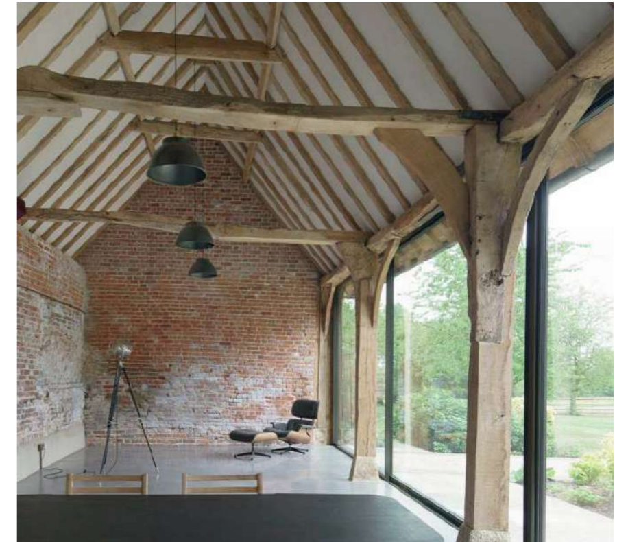
Above: The Hall - Grade II* Listed - Extensive repair, renovation & extension complete
