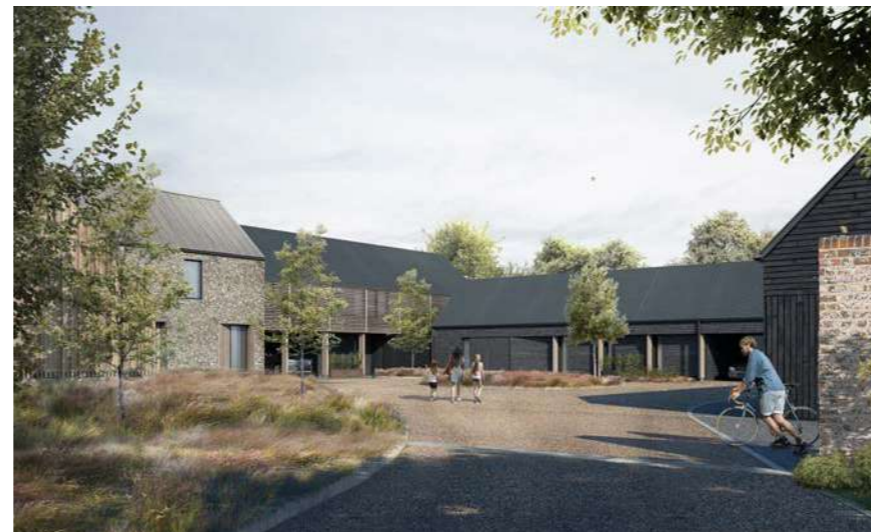
Above: Bossingham Farm (In Construction) - Conservation Area & Kent Downs AONB
