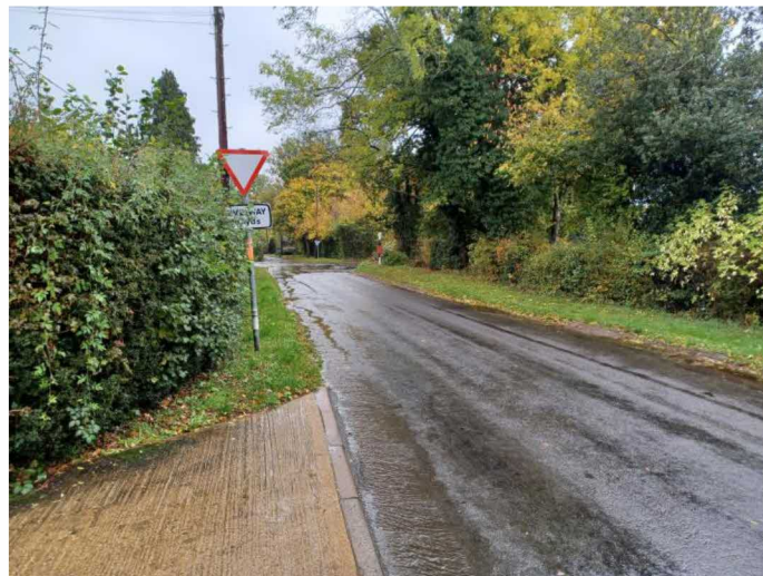
View looking east along Shantock Lane with the extended vehicle parking area to the left
