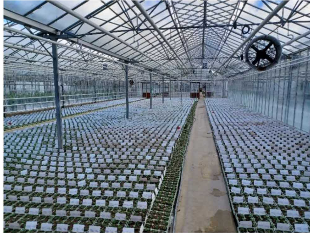
Existing production facilities at Water Lane in one of the 108 production glasshouses
