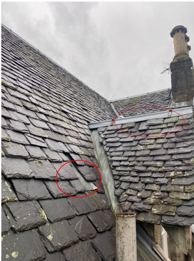
5. Rear. West facing elevation.
