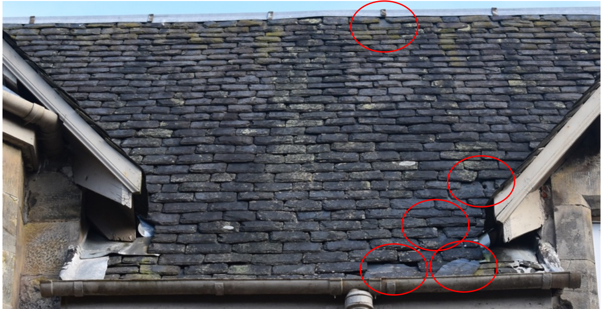
4. West facing elevation. Close-up view
