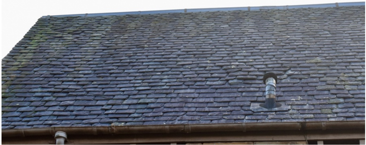
2. Close-up. North facing elevation.
