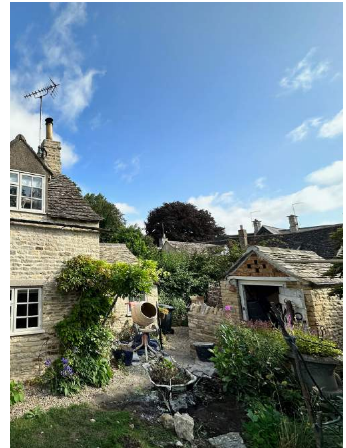
Left hand side of outbuilding (collapsed structure has been cleared away)
