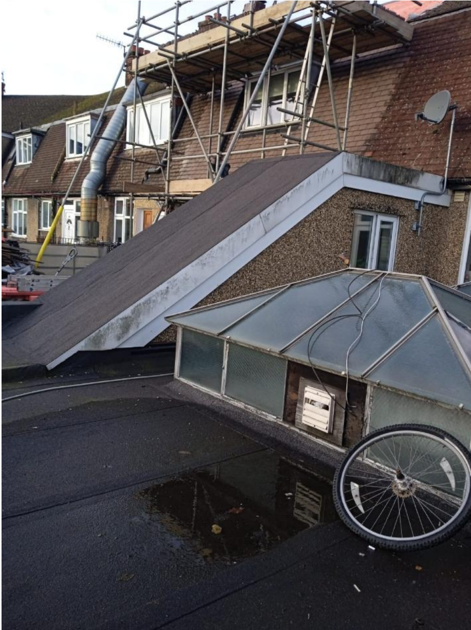
A covered stair leading to the first floor at the rear of 29 The Broadway, Darkes lane, Potters bar EN6 2HX
