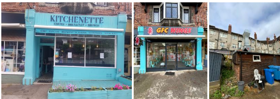
Figure 4 - The former and current shopfronts, and current rear ducting
