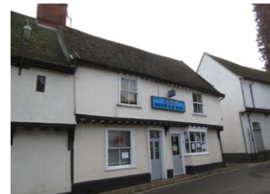
Left: looking NE showing SW gable elevation of 2 Bridge Street and entrance to yard behind the former Bull Inn; Centre: detail of SW elevation showed pargetted panels on lower part of wall of the house and shop with boarded rear range behind; Right: looking SW from Bridge Street, showing jettied front elevation of the pair of listed houses
