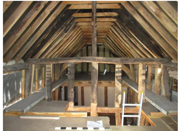
Left: looking W from SE bay showing 3 crown posts with original collar purlin beneath replacement collars; Right: looking NW from SE loft showing open framing with lath marks beneath SE crown post
