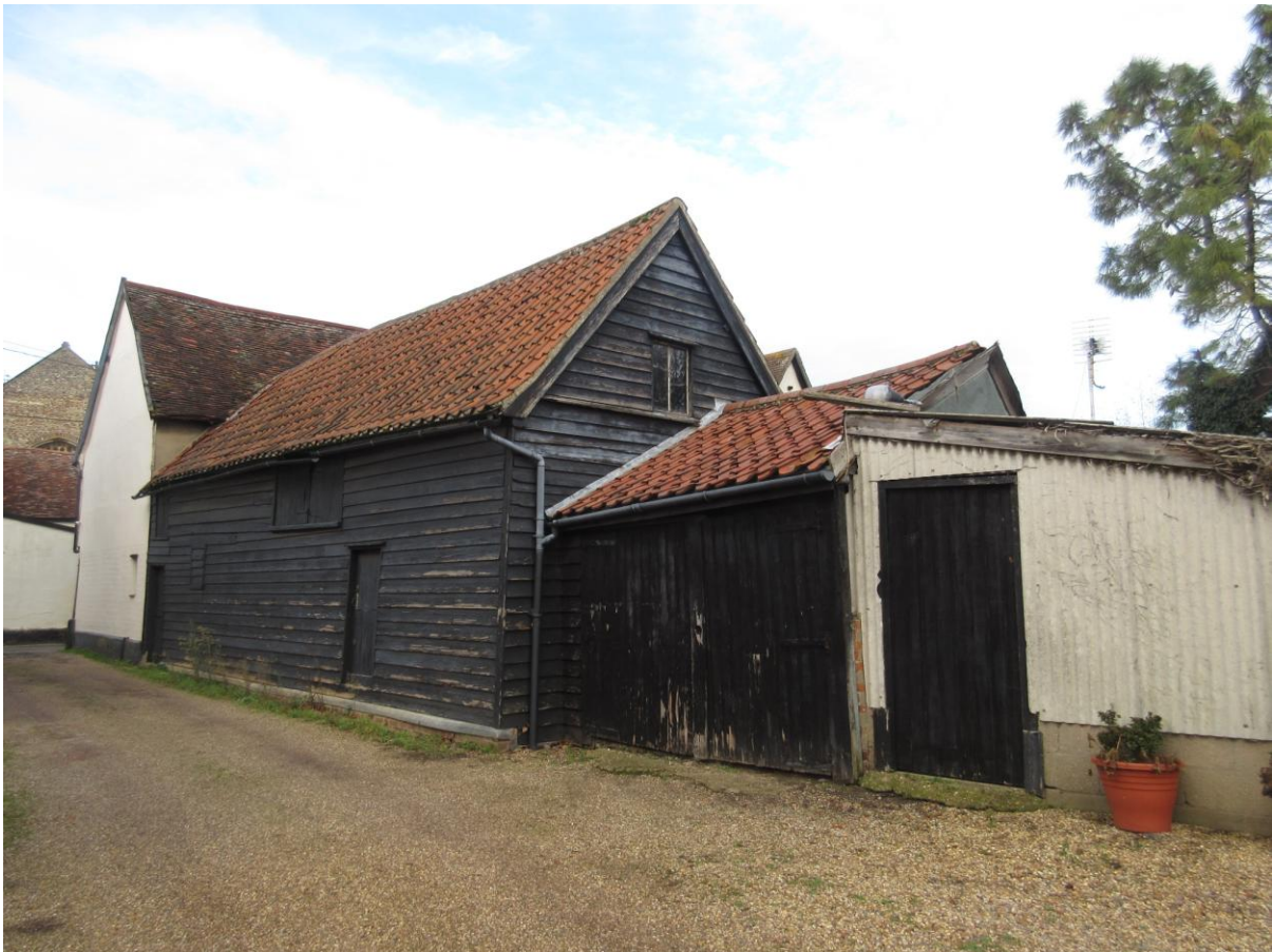
Rear range attached to 2 Bridge Street, looking NE
