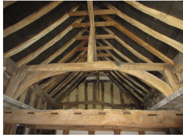
Left: NW crown post next to SE wall of 2 Bridge Street, looking W, showing cranked tiebeam; Right: looking NW from ground floor of middle bay showing massive binding beam with empty joist mortices, tiebeam above with crown post between NW and middle bays
