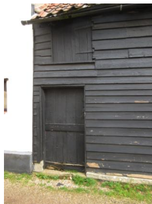
SW Elevation: Left: former stable door in SE bay showing common brick plinth with lead covering; Centre: former stable door and loading door in NW bay; Right: former loading doors between middle and SE bays showing strap hinges
