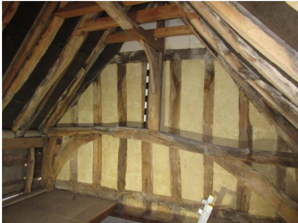
Left: NW crown post next to SE wall of 2 Bridge Street, looking W, showing cranked tiebeam; Right: looking NW from ground floor of middle bay showing massive binding beam with empty joist mortices, tiebeam above with crown post between NW and middle bays
