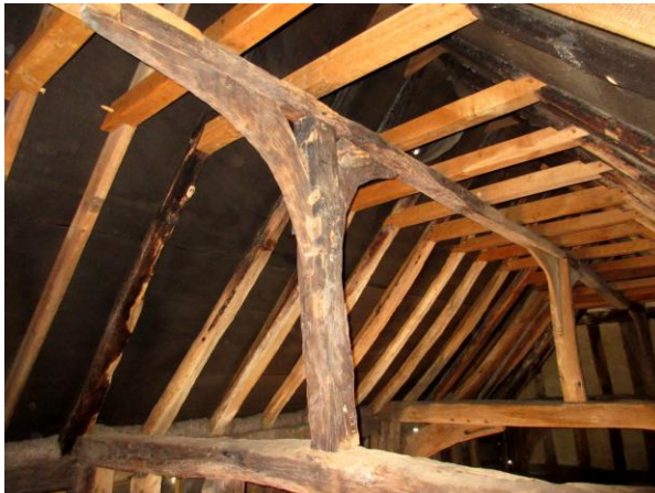
Left: looking W from SE bay showing 3 crown posts with original collar purlin beneath replacement collars; Right: looking NW from SE loft showing open framing with lath marks beneath SE crown post
