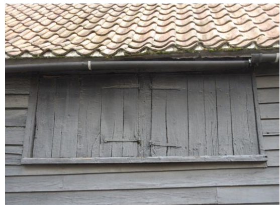
SW Elevation: Left: former stable door in SE bay showing common brick plinth with lead covering; Centre: former stable door and loading door in NW bay; Right: former loading doors between middle and SE bays showing strap hinges
