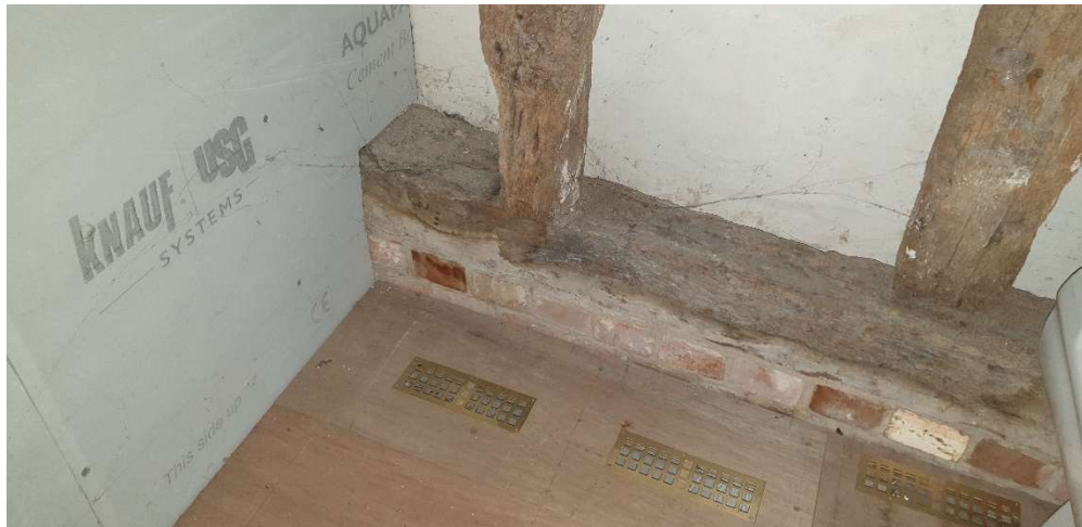
Ground floor as installed, uninsulated, and wall lining
