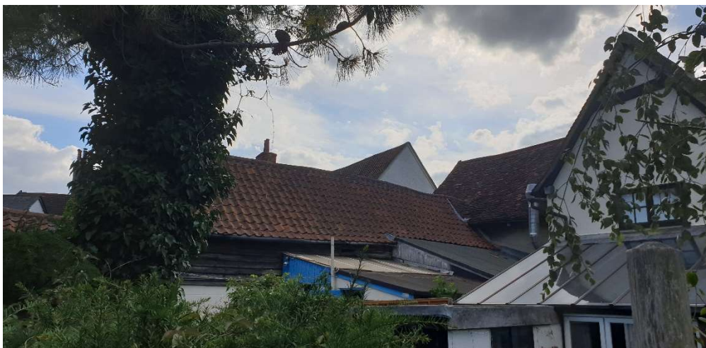
Northern wall of the barn with adjacent lean to structures
