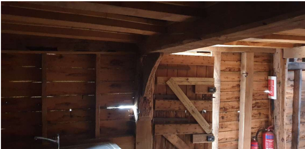
Existing south wall
