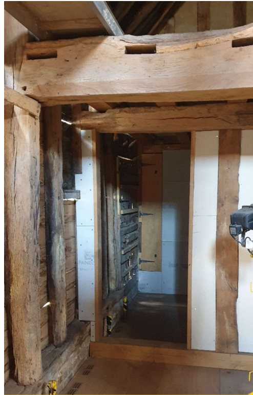
Image of the roof interior looking west, illustrating repaired and replacement timbers, and new floor as inserted
