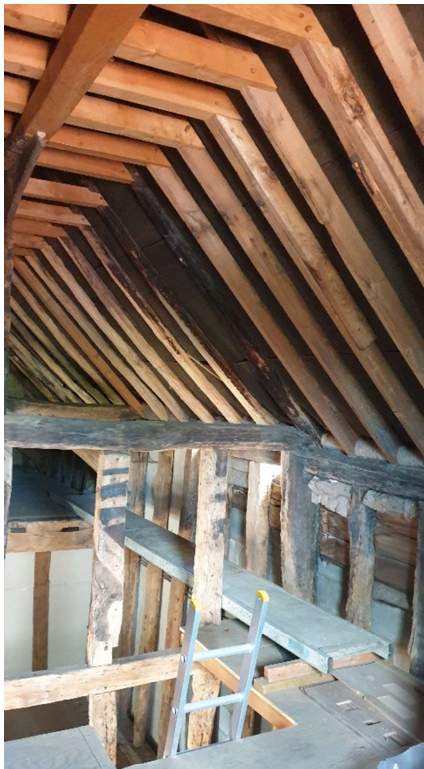
Image of the roof interior looking west, illustrating repaired and replacement timbers, and new floor as inserted
