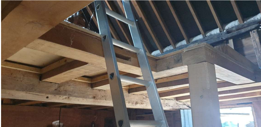
Floor / stairwell as installed
