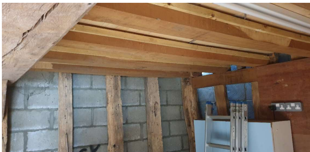
Existing northern wall, with blockwork compartment wall to adjacent lean-to structures
