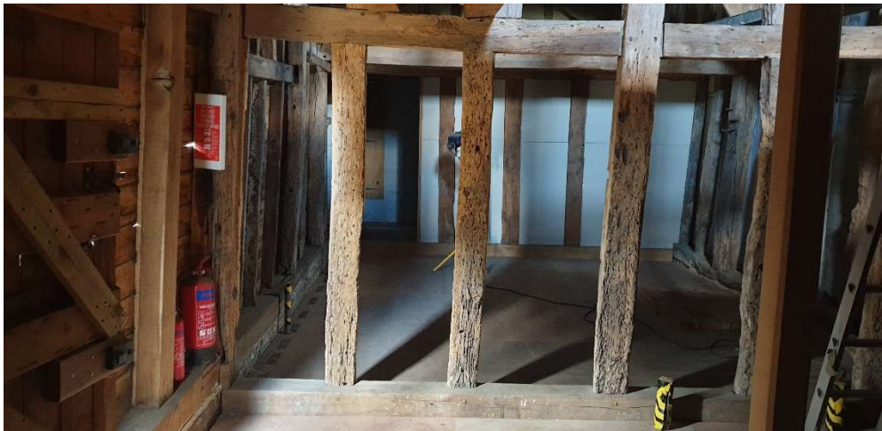
Stud and plate to be removed for access
