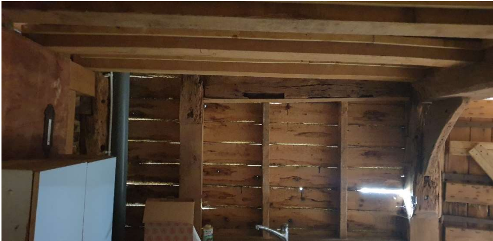
Existing south wall where approved window to be cut in
