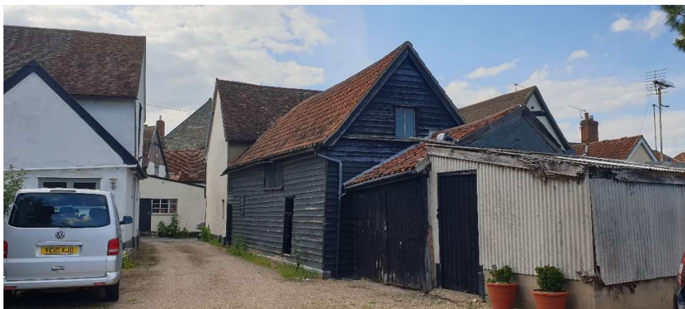
Barn viewed from the south east, looking towards Bridge Street
