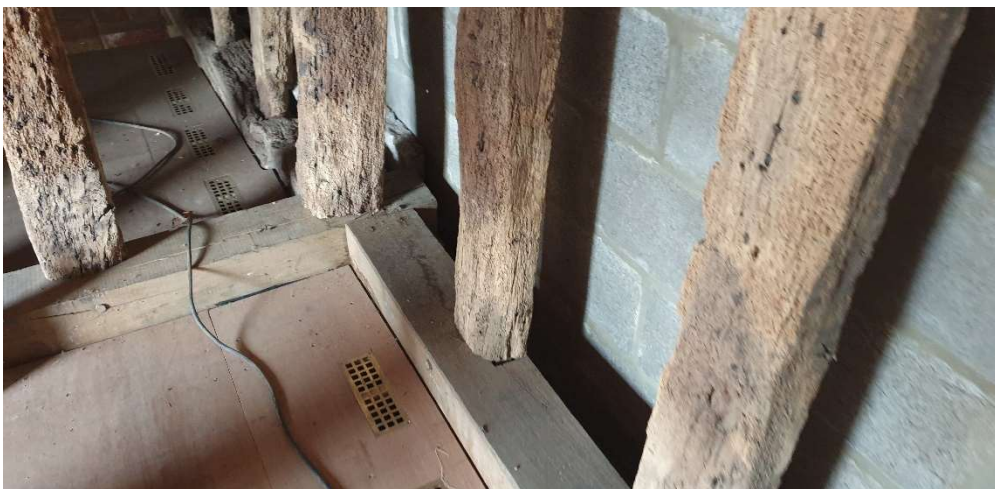
Replacement sole plates, and northern blockwork wall
