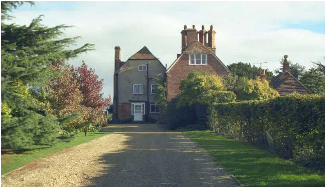
Fig. 10: View, looking south-east, of the north-west elevation of Tadley Place Farmhouse, with the eighteenth-century addition to the right (Historic England).
