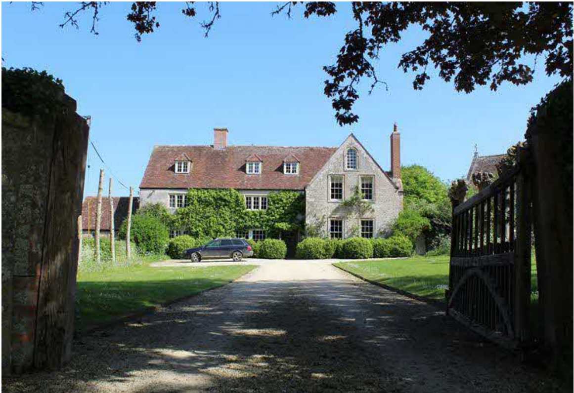
Fig. 21: The principal, south elevation of Hill Deverill Manor (Historic England).
