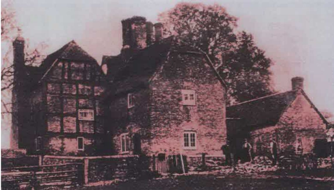
Fig. 13: An early twentieth-century photograph of the north-west elevation of Tadley Place Farmhouse, with exposed timber box-framing on the left-hand side (Forum Heritage Services Ltd).
