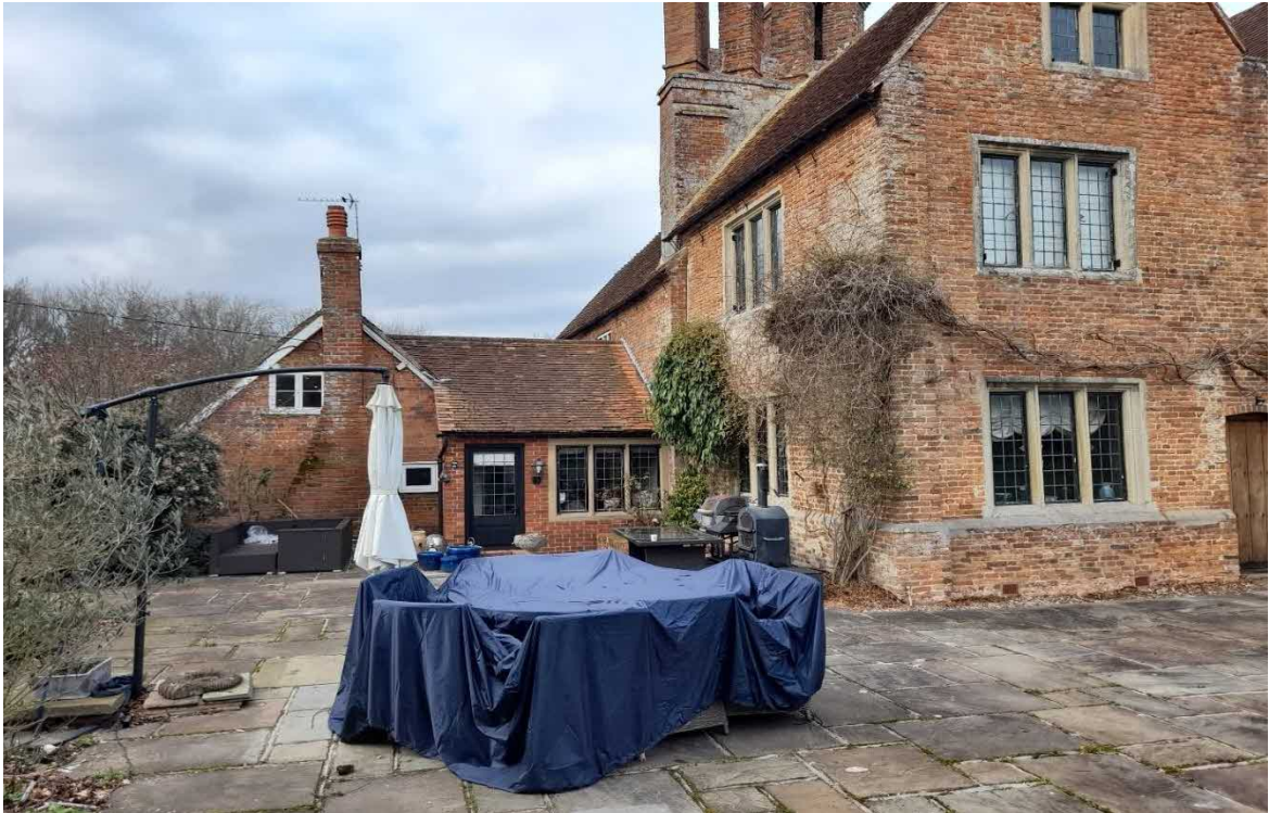
Fig. 6: View, looking north-west, of the left-hand gable of the south-east, front elevation, and the south-west elevation.
