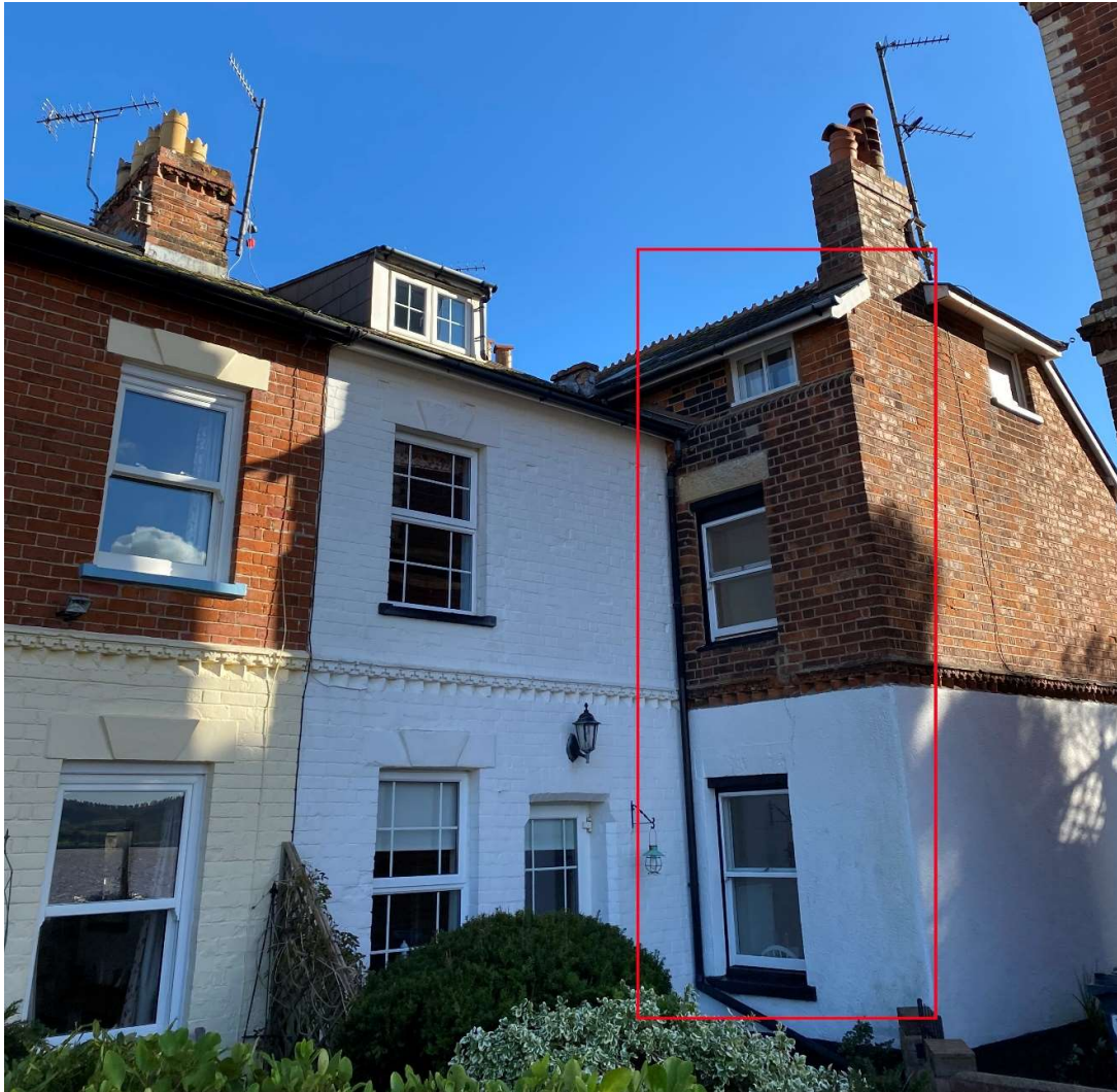
Photograph 3: Red line identifies existing windows that enable occupiers to view the private amenity spaces of adjoining dwellings. The photograph also shows the inconsistency in the style and material of windows; timber frames and uPVC frames.
