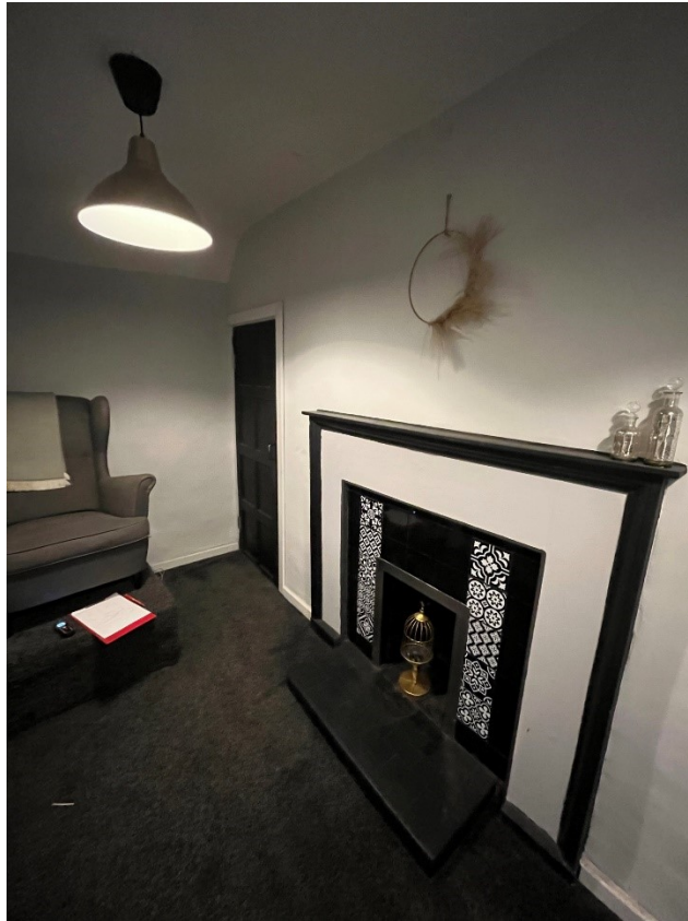
5. 17 th century wainscot door and adjacent fireplace in rear first floor room, now partitioned to form a lobby, kitchenette and WC.
