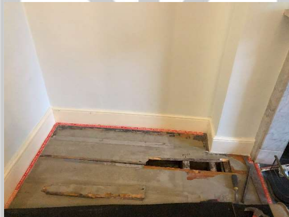
Floor structure in proposed location
