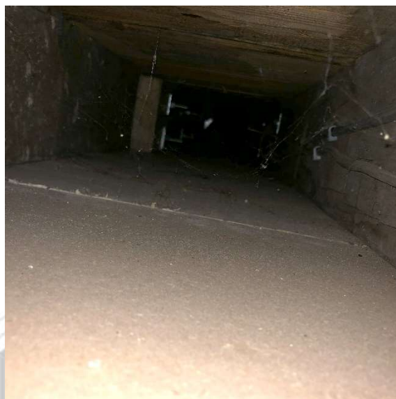
Ground Floor structure with previous repair works just visible
