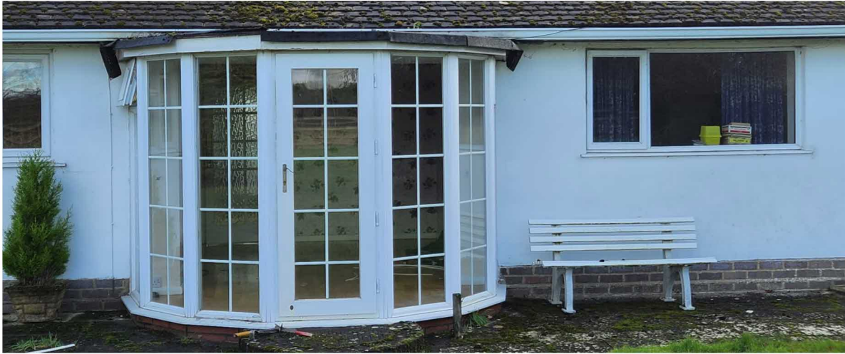
Fig.3 – Previous photograph of rear elevation showing bay window
