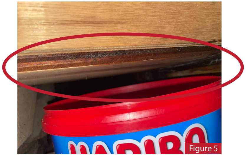
Water ingress onto existing lay-board
