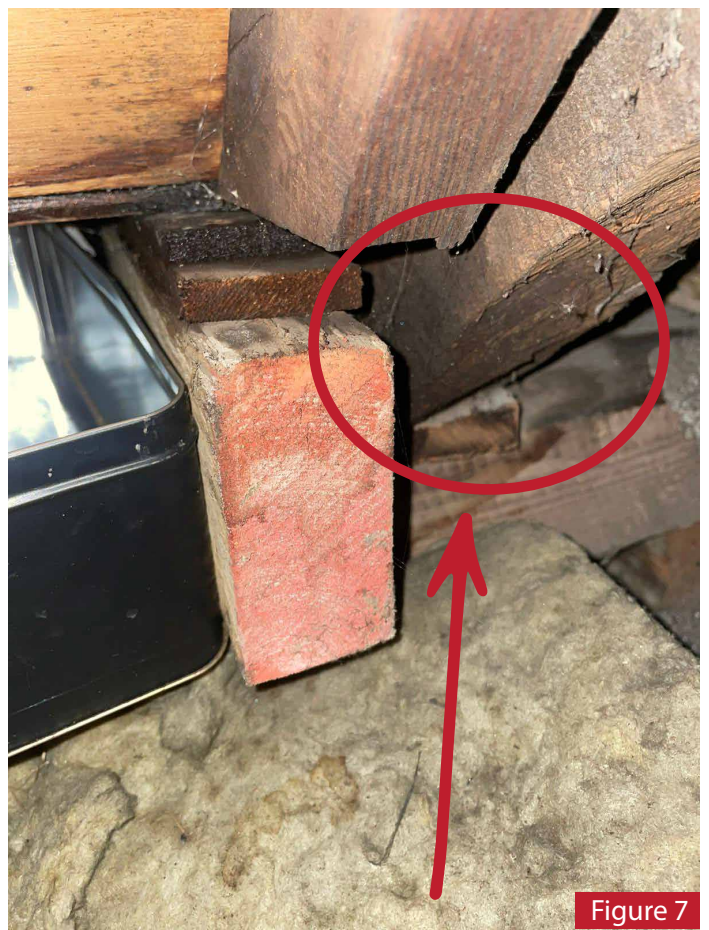
Evidence of water damage resulting from an extended period of leakage.
