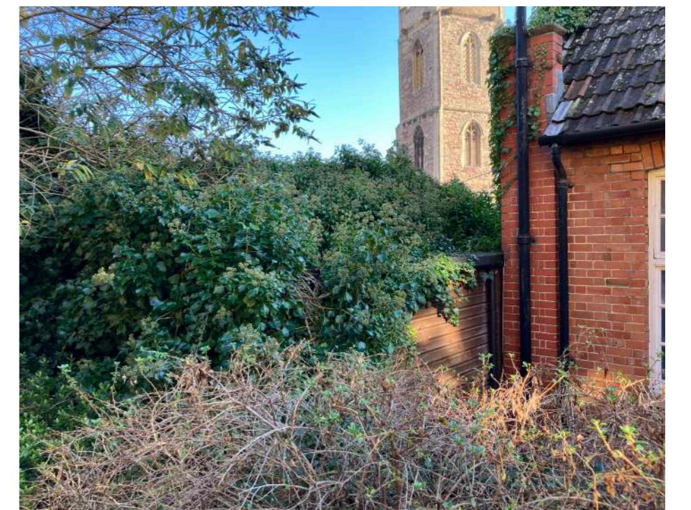
Existing scrub on the roof of the existing scout hut.
