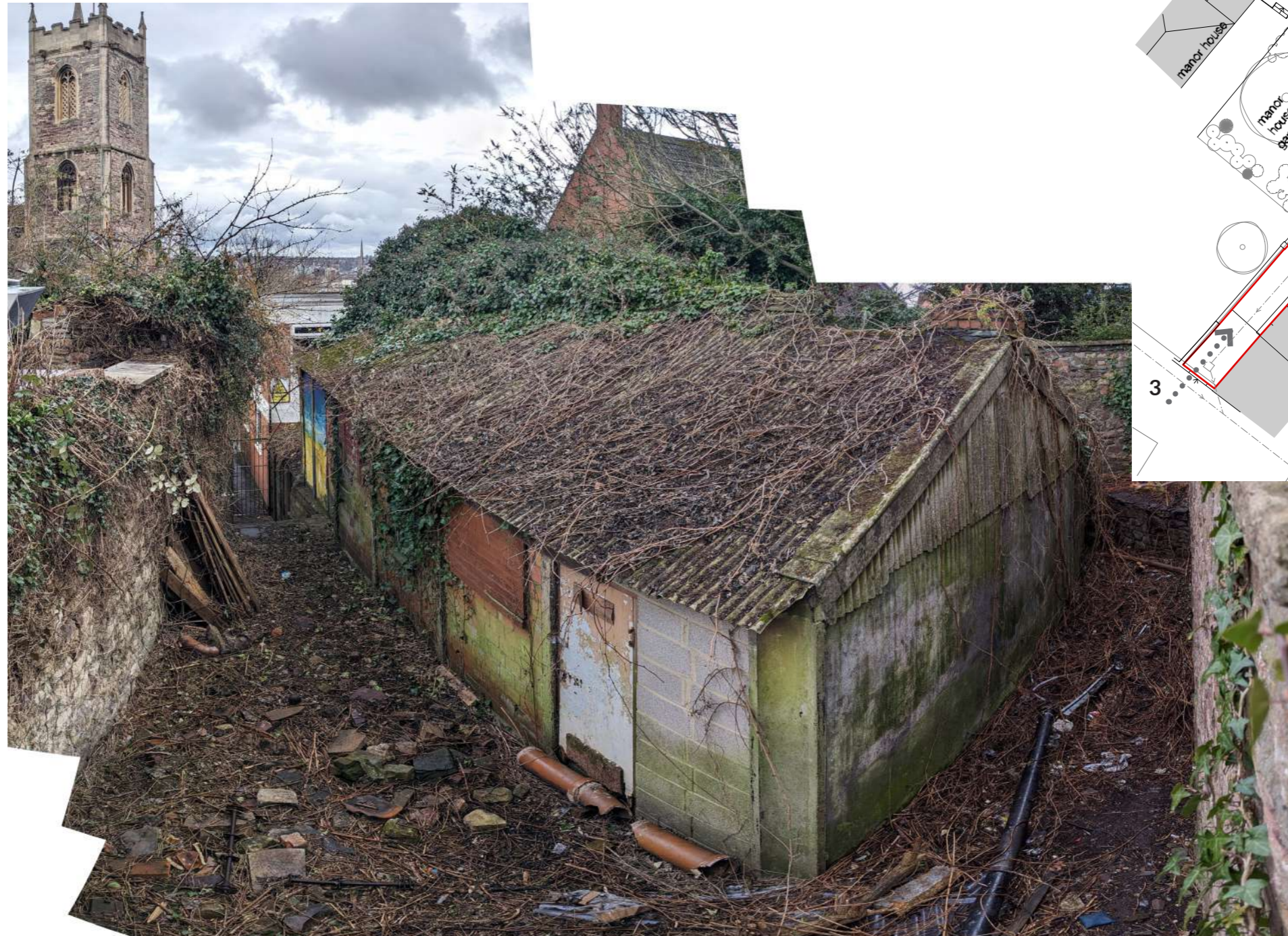
4. Existing site looking SE from Mansion House terrace
