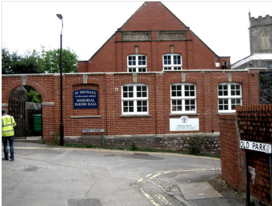
3. Image showing the south-western gable end of the Memorial Hall building, with its inscription above the upper set of windows reading 'St Michael's Parish Hall'. View to north-east.
