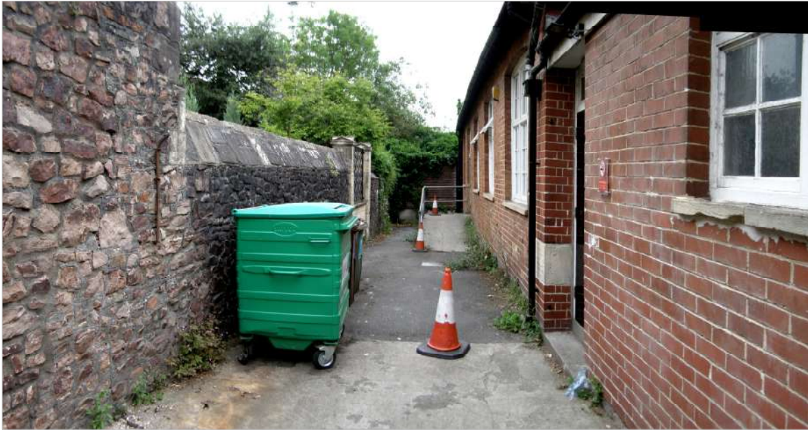
5. The narrow alleyway separating the north-western elevation of the Memorial Hall (right), from the Manor House's south-eastern boundary wall (left). Note the gate pillars about halfway along the masonry wall, marking the now-blocked original access into the lower garden belonging to the Manor House, the site of which was later occupied by the Memorial Hall. The blocking is most likely to have occurred at the same time as the construction of the Memorial Hall. View to north-east.
