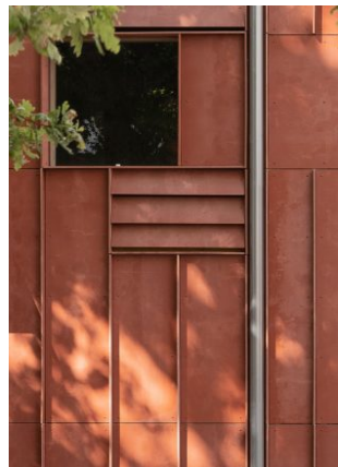
Example cladding: Viroc composite panel cladding and reveals to windows (4)
