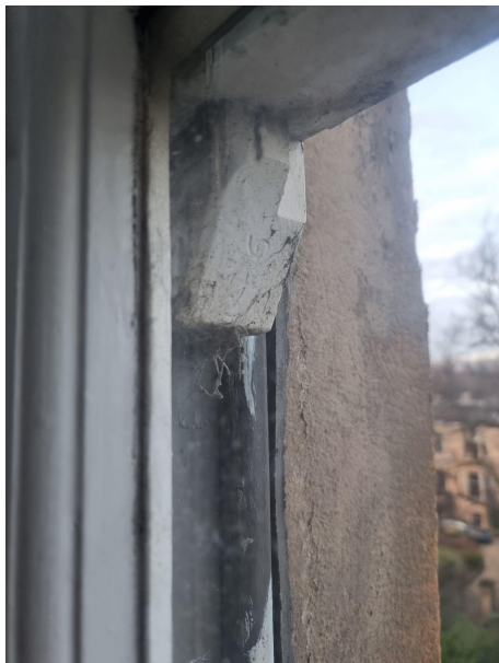
Further photos of the dead horns to windows on the front elevation, along with sharp moldings to the sashes internally.
