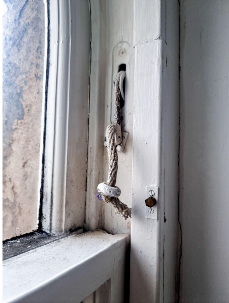
The first photo shows a broken rope and pulley wheel. The second photo shows a “dead horn”, this shows that the window is not original as the horn does not match the windows on the lower floors of the building. There are also sharp moldings to the windows which show they are not original windows.
