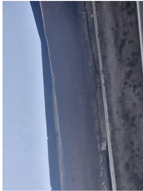
Rotting midrail woodwork.
