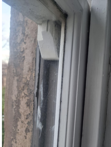
The first photo shows a broken rope and pulley wheel. The second photo shows a “dead horn”, this shows that the window is not original as the horn does not match the windows on the lower floors of the building. There are also sharp moldings to the windows which show they are not original windows.
