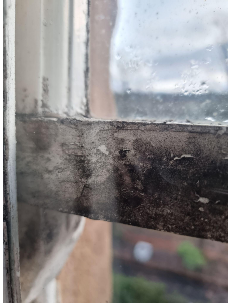
Rotting midrail woodwork.
