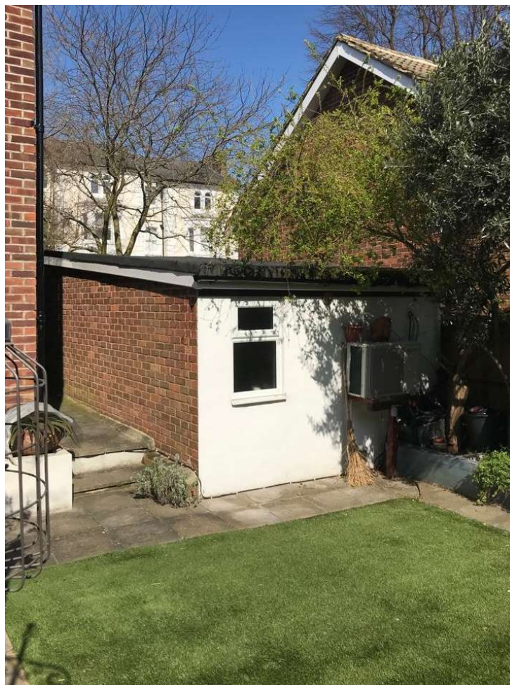
01 Image: Photograph of Application Site (Existing Studio)
