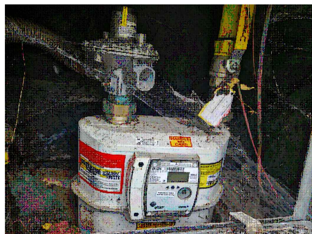
EXISTING GAS METER KIOSK/HOUSING LOCATION AT SITE BOUNDARY
