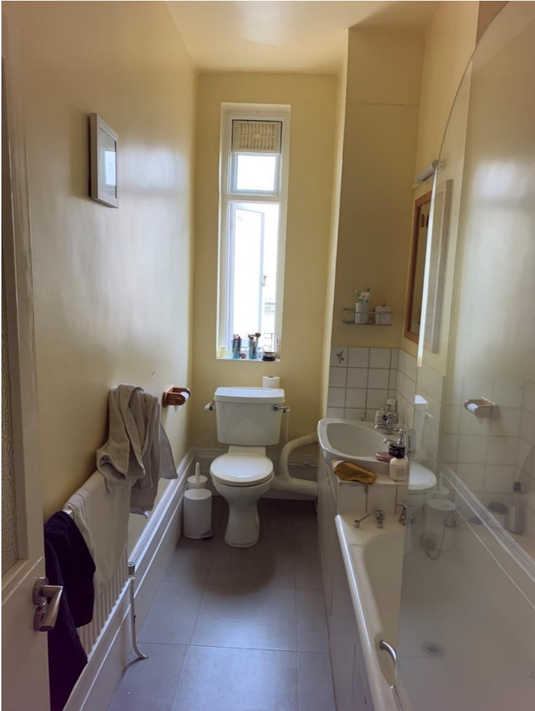
Figure 11 Existing Bathroom showing dropped ceiling and partitions
