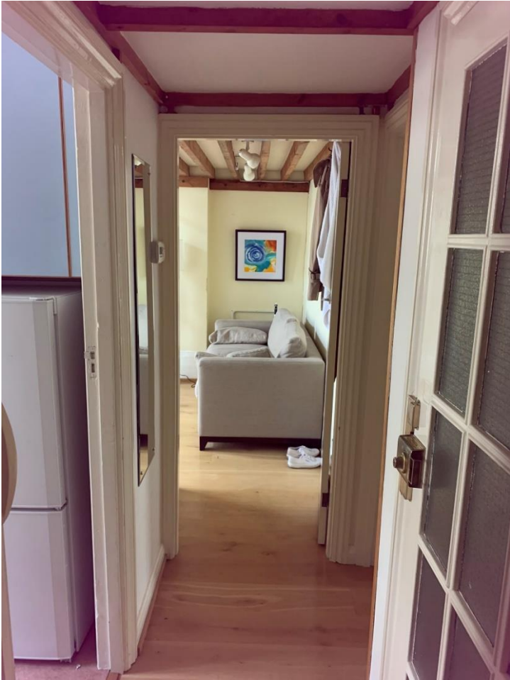
Figure 9 Existing hall showing dropped ceiling
