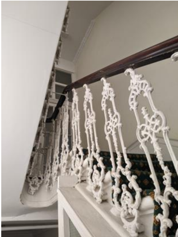
Figure 6: Stairwell with decorative cast iron spindles and polished hardwood handrail.
