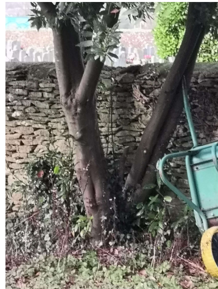
Bay has multiple trunks. Again the right hand side trunks are likely to be removed to reduce risk to the integrity of the dry stone wall.
